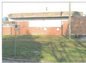
2. CONTEXT STREET VIEW - SOUTH
