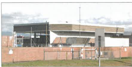
1. CONTEXT STREET VIEW - SOUTHWEST
