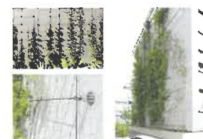
Metal lattice system for vines to grow up building facade
