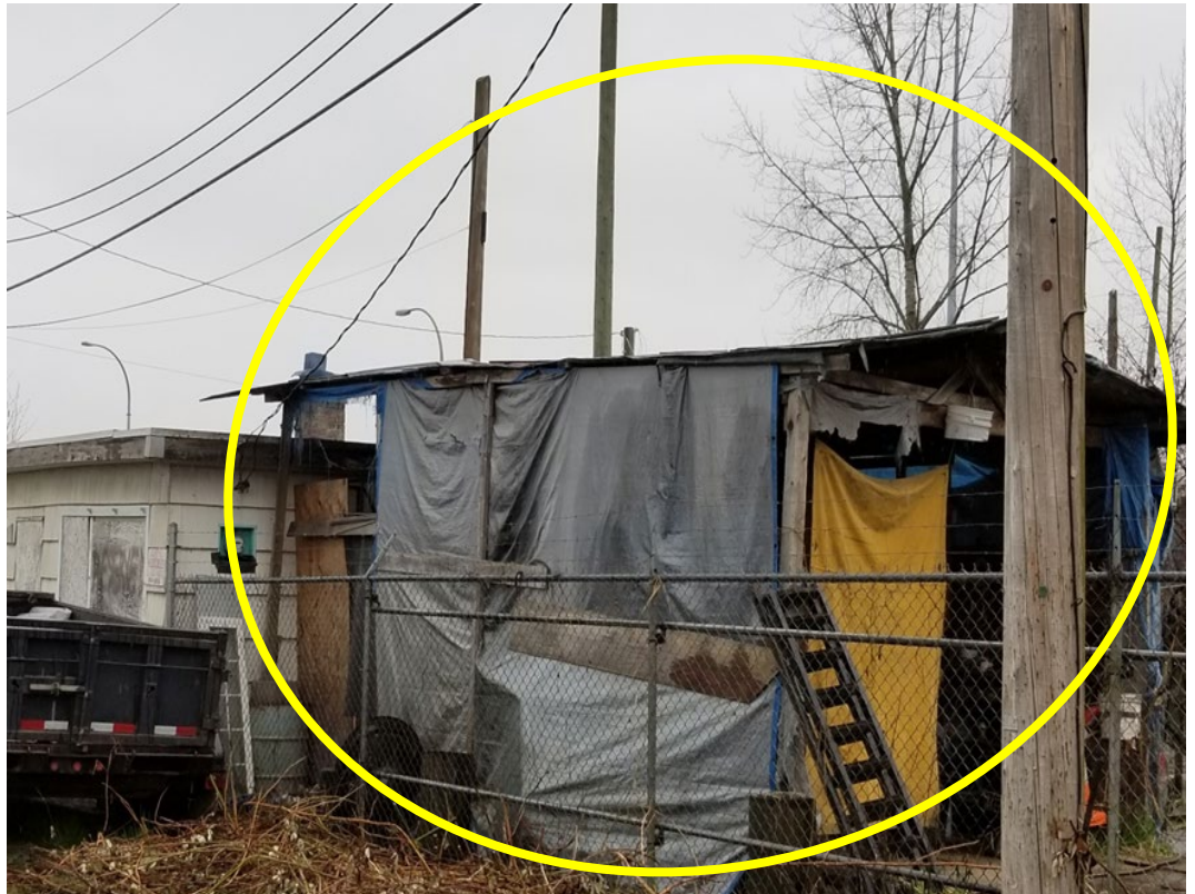
Photo 1.1 Addition without a permit – Structurally unsafe
