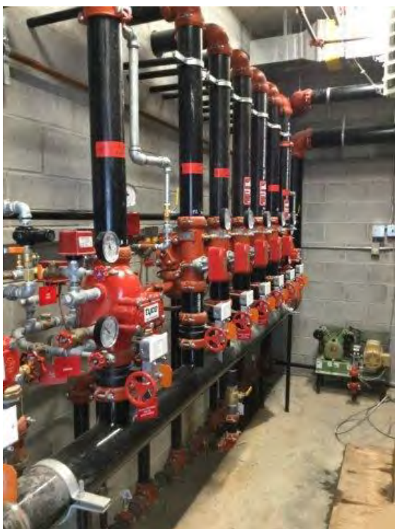
Phase 1B – Sprinkler tree ready for labelling
