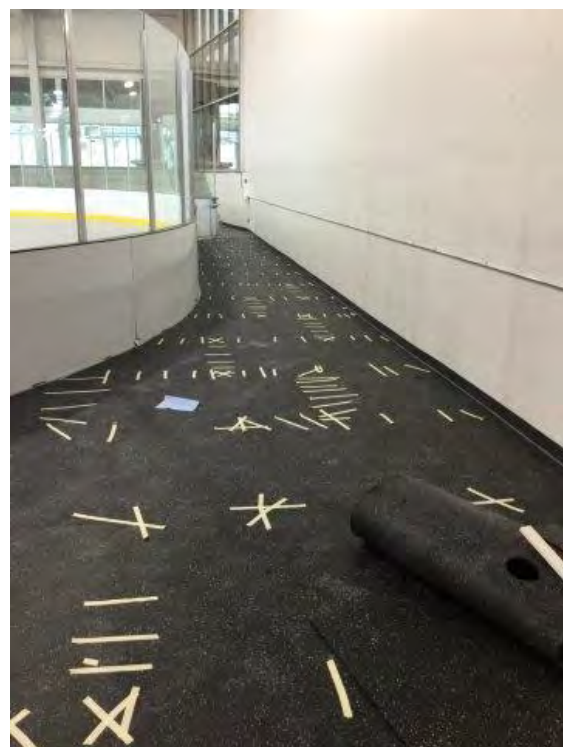
Phase 1B – Rubber skate flooring install
