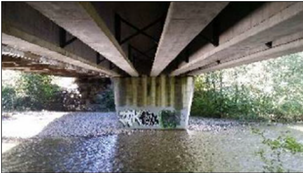
Figure 5: Existing pier of westbound concrete bridge
