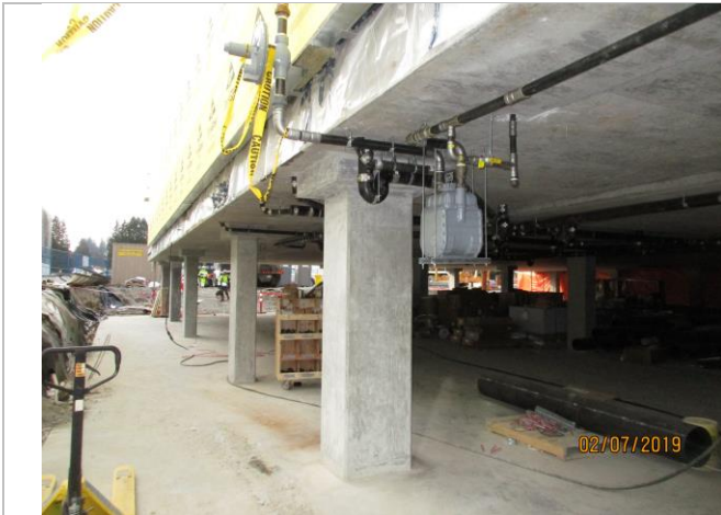
Photo #5: Temporary Gas Meter
