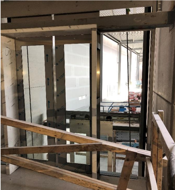
Elevator 2 Level 2 frame installation.
