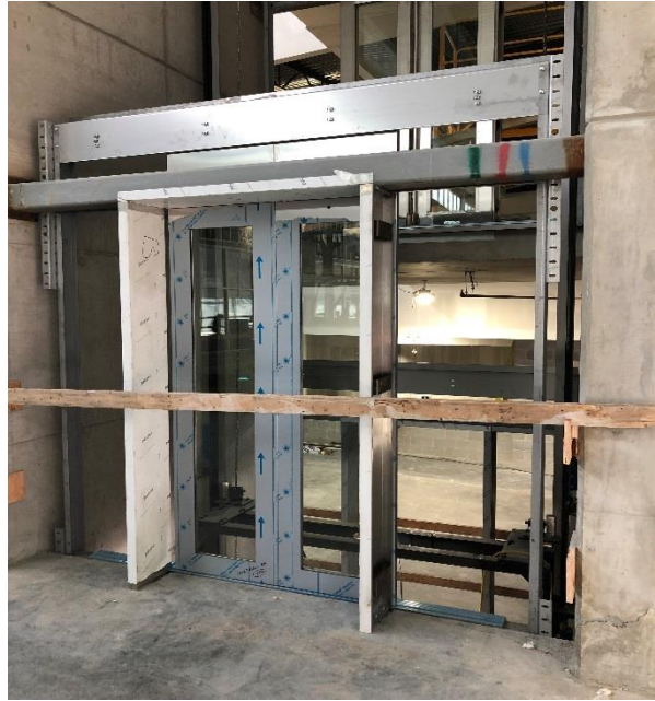
Elevator 2 Level 1 frame installation.
