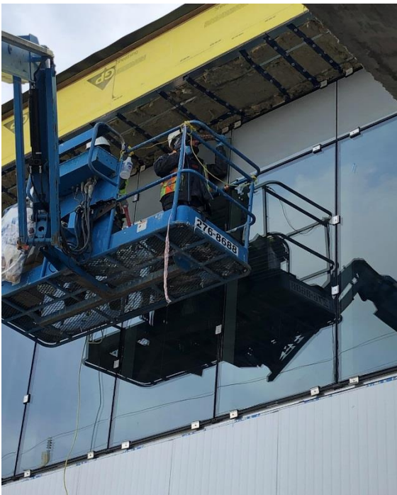
Rink 3 north face Spandrel glass sealant.
