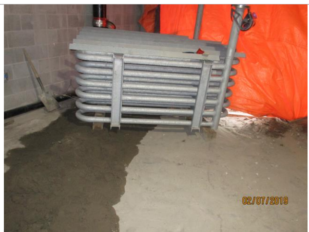
Photo #10: Ice melt pit coil
