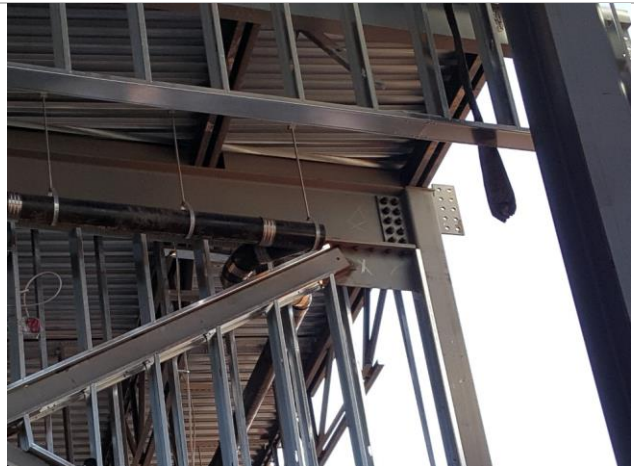
Photo #11: P2C, Level 2: Storm drain piping in ceiling
