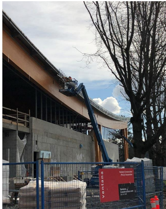
Phase 1C west face roof parapet framing
