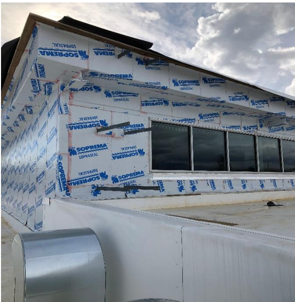
Public Corridor 1B118 north exterior wall GL 1B-F AVB. Wall type W5
