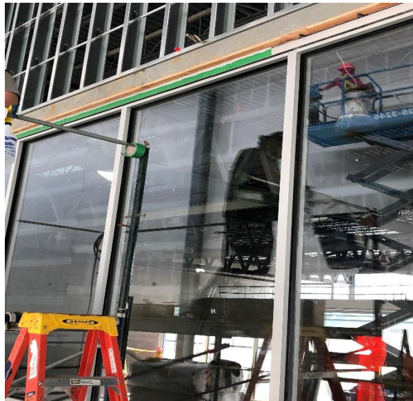
Public Corridor 1B118/Rink 3 along GL 1B-F mullion frame joint sealing.
