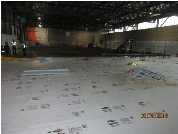
Photo #1: Rink #3 Slab Insulation
