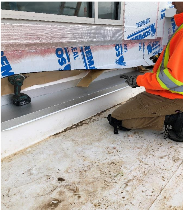
Public Corridor 1B118 north exterior wall GL 1B-F pre-finished metal flashing. Wall type W5
