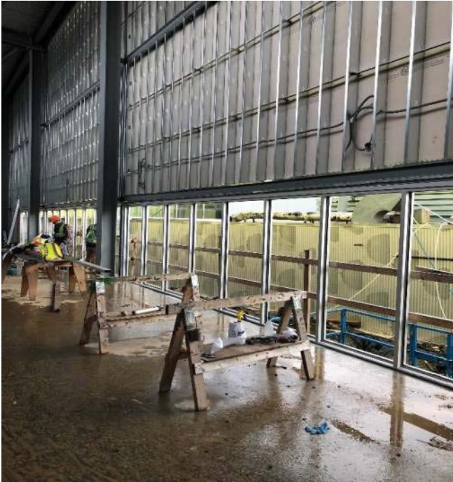
Public Corridor 1B118 south elevation mullions.
