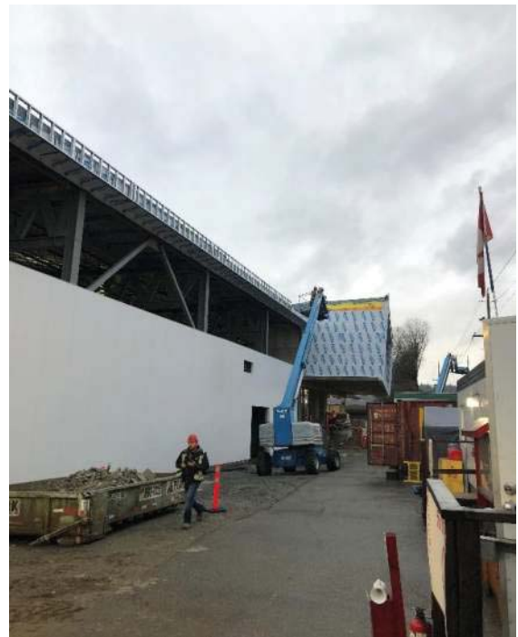
Rink 3 north elevation parapet framing.
