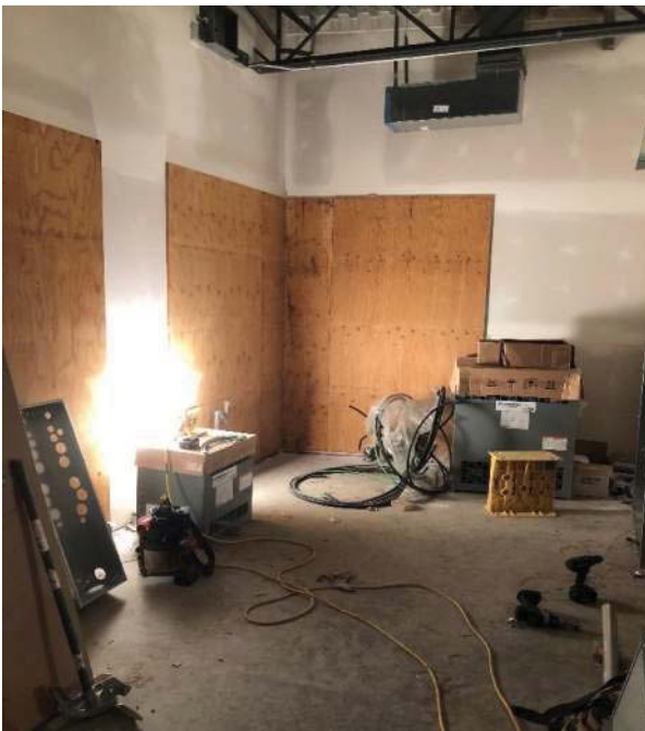
Phase 1A Electrical room 1A201 electrical panel backing.
