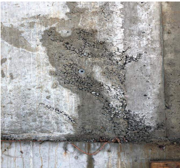
Phase 1C Level 1 to Level 2 exterior face along GL 1C-1 concrete to be repaired.
