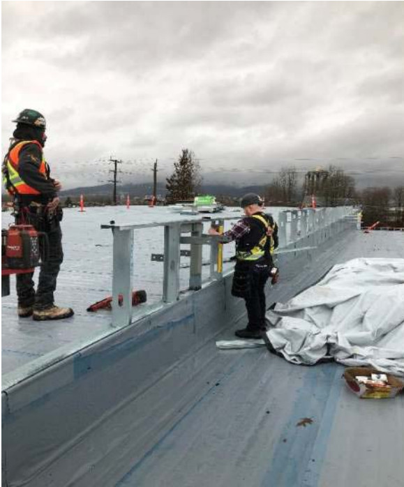
Library roof parapet framing
