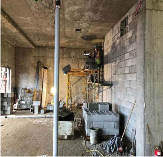
Phase 1C Level blockwalls from GL 1C-1 to 3 between 1C-D+ to J.
