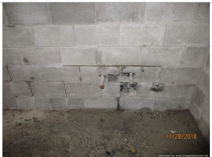
Photo 4: Piping Rough-ins for changeroom washroom fixtures in progress
