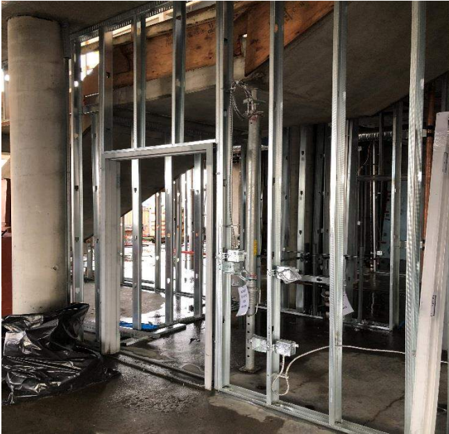
Level 1 Library steel stud framing.
