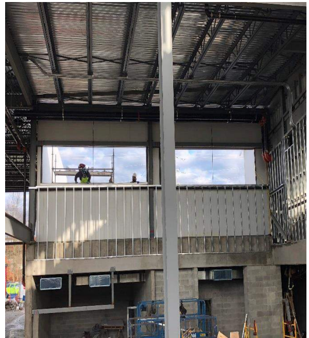
Phase B steel stud framing along 1B-E- between 1B- 11 &13
