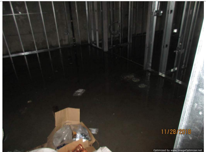
Photo 8: Some excess water pooling in the library area observed as a possible hazard to be addressed on site.
