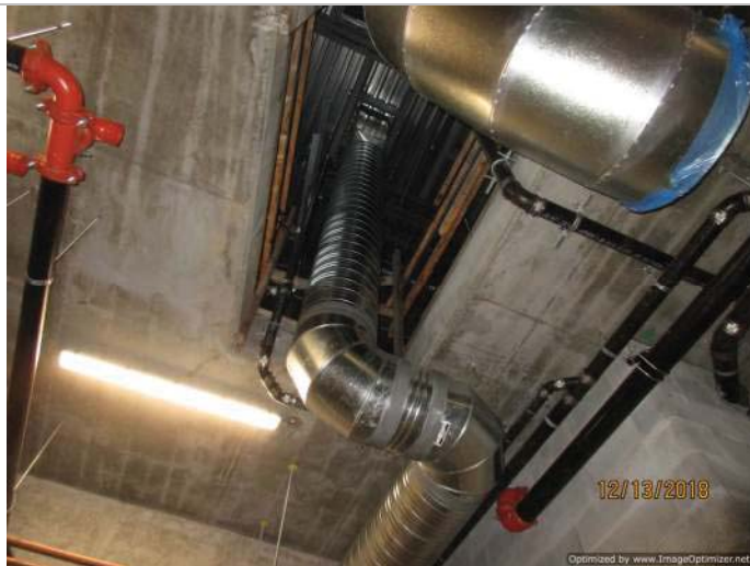
Photo 1: Exhaust Duct Riser
