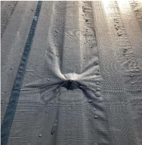
FR#19 - Rink 3 bolt protruding through AVB to be repaired. This occurs in a few locations.
