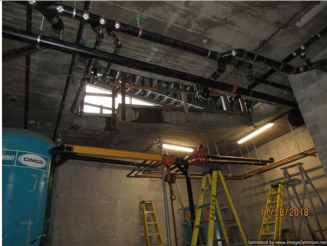
Photo 5: Sanitary piping in refrigeration room ceiling serving concession fixtures above. A portion of the ceiling is open for future mechanical service shaft install.
