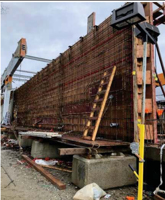
Phase 1C Level 1 to 2 wall formwork and reinforcing along GL 1C—1 between 1C-J & 1C-P.
