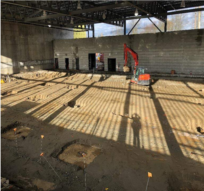
Rink 3 pile cap excavation
