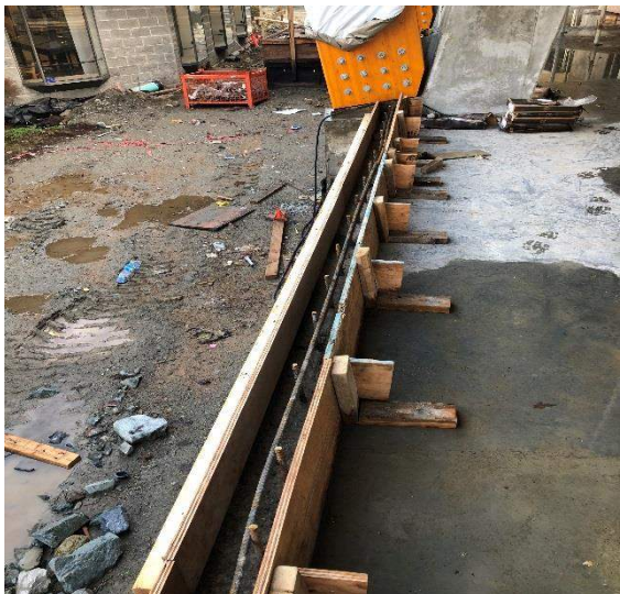
Phase 1C curb formwork along gl 1C-A
