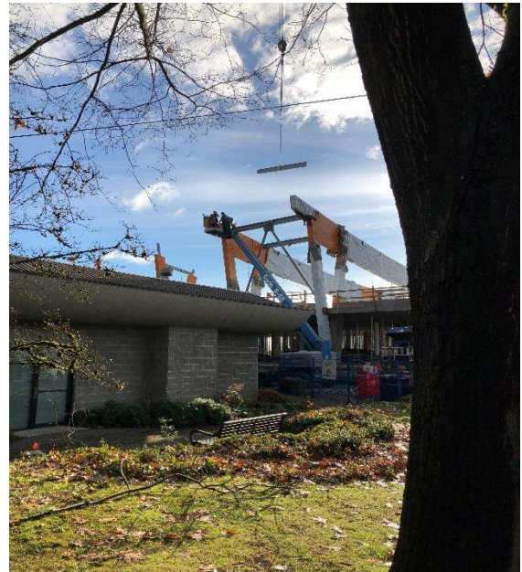
Phase C Glulam structural bracing installation looking southeast.
