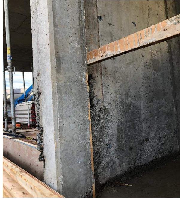
Phase 1C Level 1 to Level 2 interior face along GL 1C-C Stair 1C3 concrete to be repaired.
