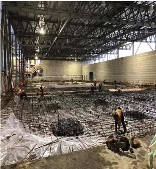
Rink 3 slab reinforcing.
