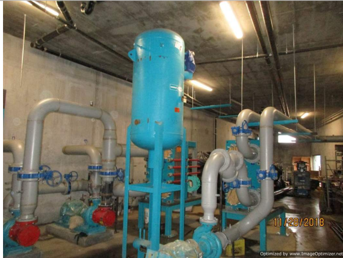
Photo 11: Refrigeration Room equipment and piping installation in progress
