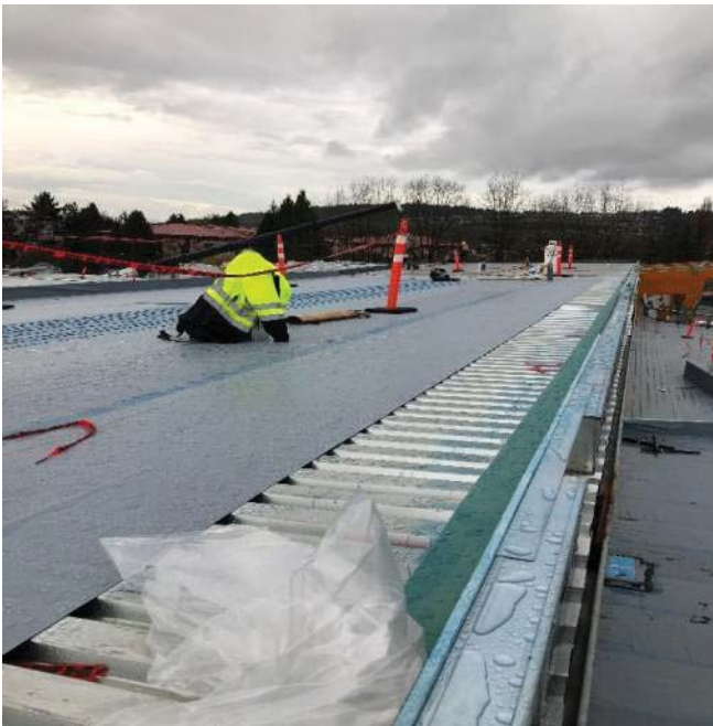
Public Corridor roof AVB installation.
