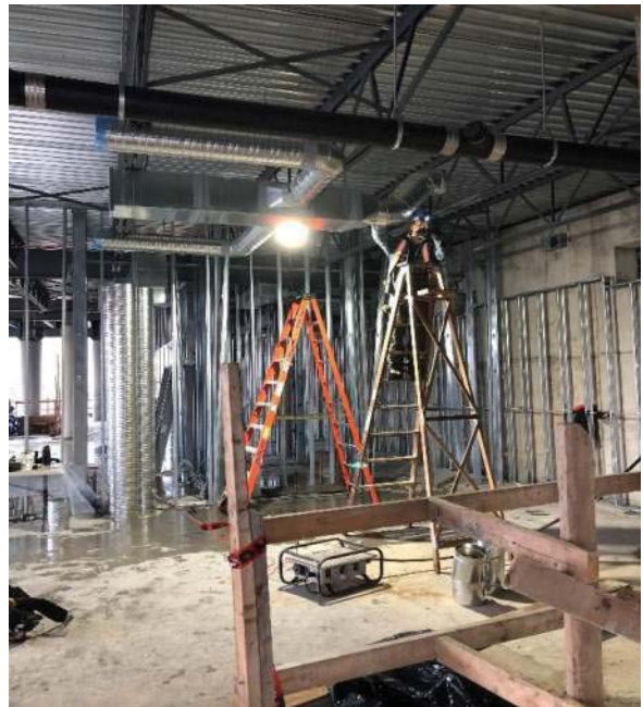
Level 2 Library ducting installation
