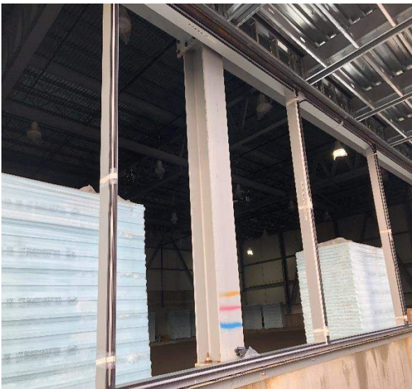
Rink 2 east elevation glazing framing
