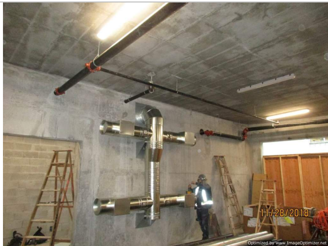
Photo 1: Sheet metal ducting and piping inside Ice Resurface Room in progress
