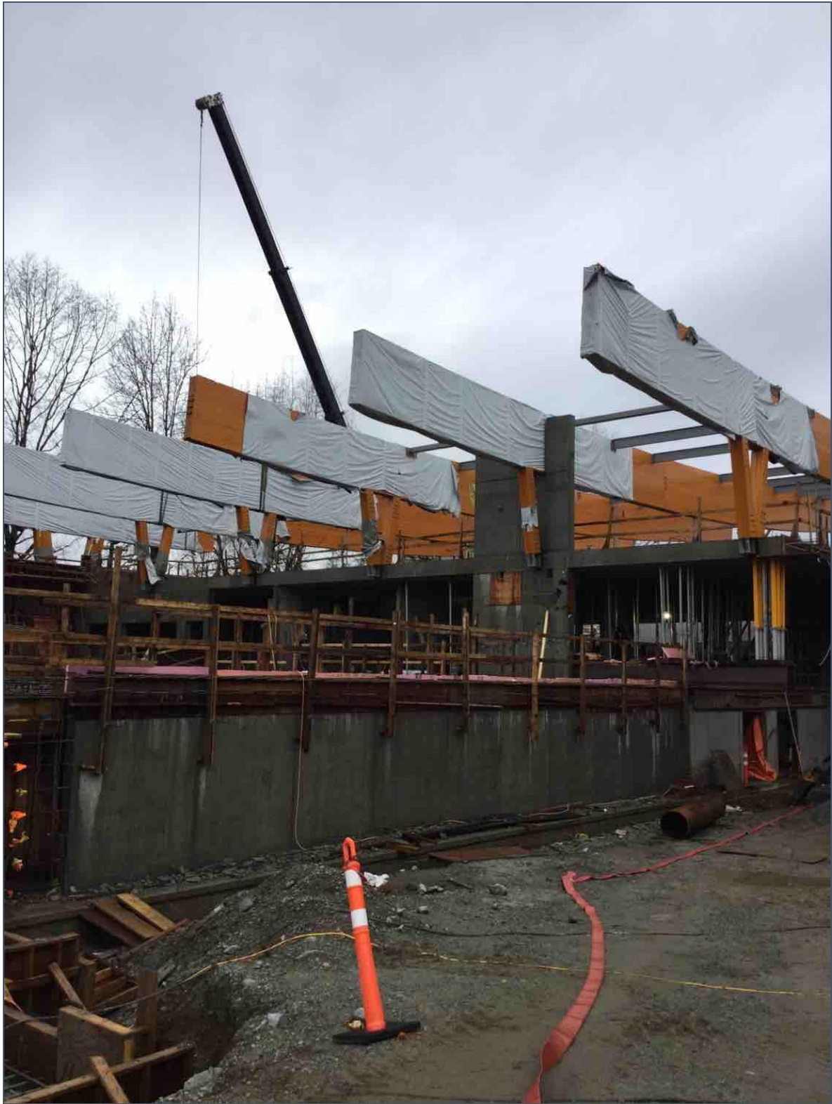
Phase 1C – Glulam installation
