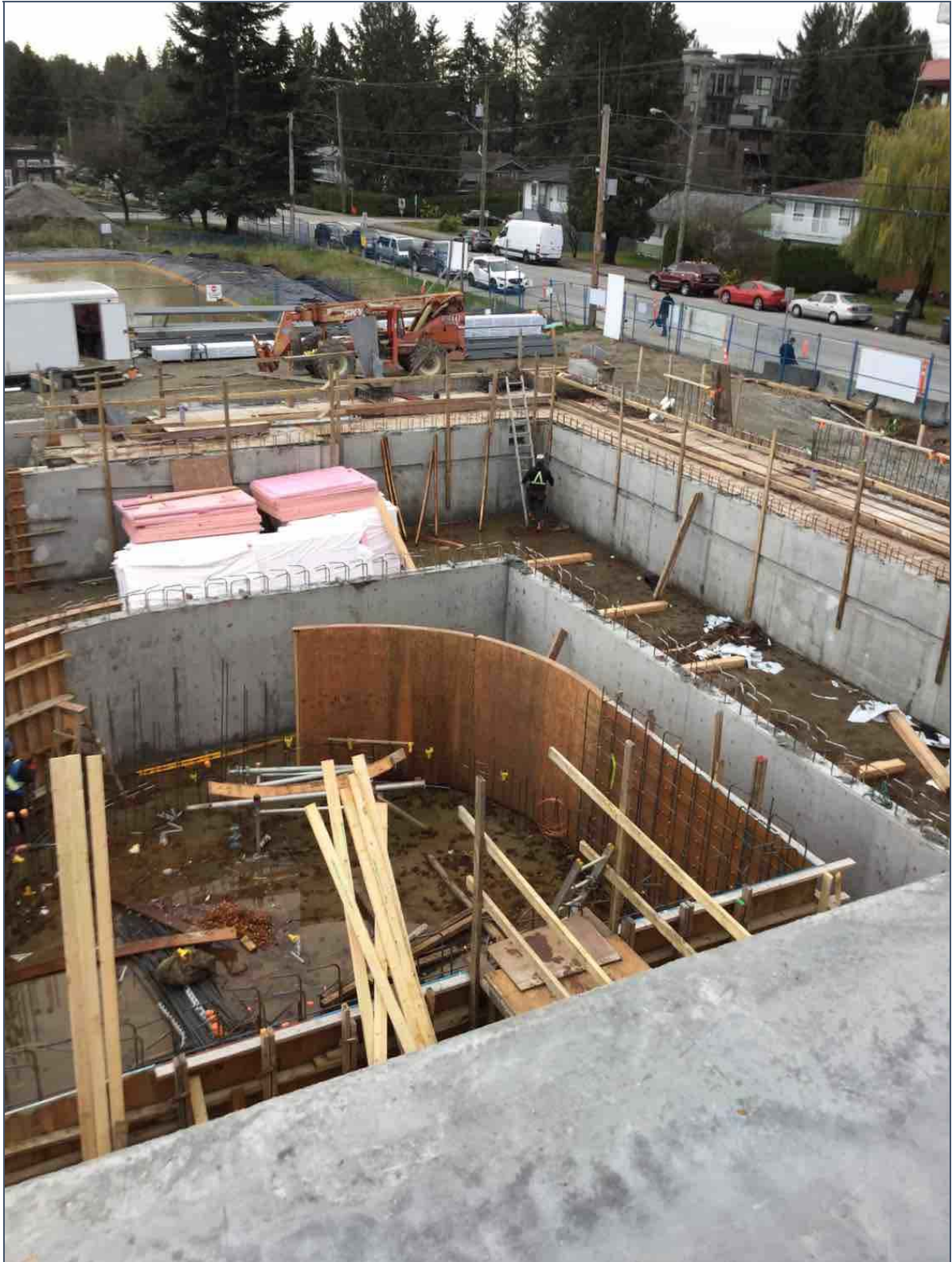
Phase 1C – Lap tank and hot tub wall formwork progressing
