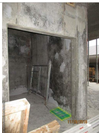
Photo 9A: 150mm storm piping at public corridor for phase 1C. Photo 9B: Marked RWL drop in room 1C120 appears to conflict with door entry.
