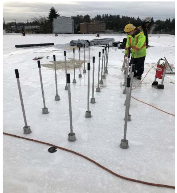
Rink 2 roof membrane welding.
