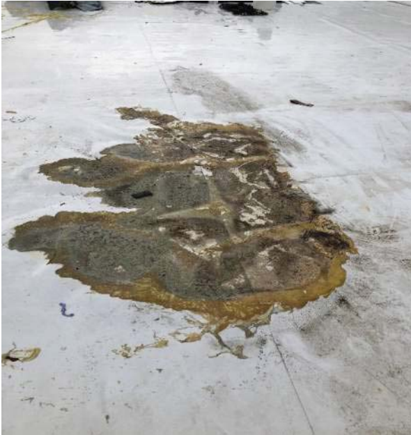
Rink 2 roof. Glue to be removed and area repaired if required.
