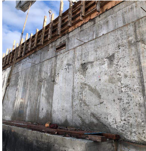
Phase 1C Level 1 to Level 2 exterior face along GL 1C-1 concrete to be repaired.
