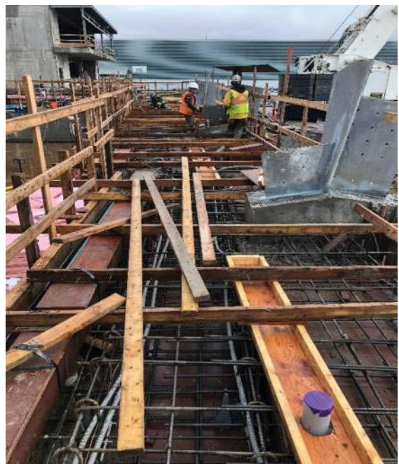
Phase 1C Level 1 Pool slab formwork.
