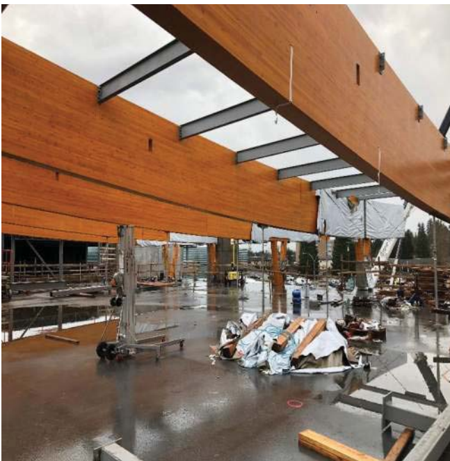
Phase C Glulam structural framing looking southeast.
