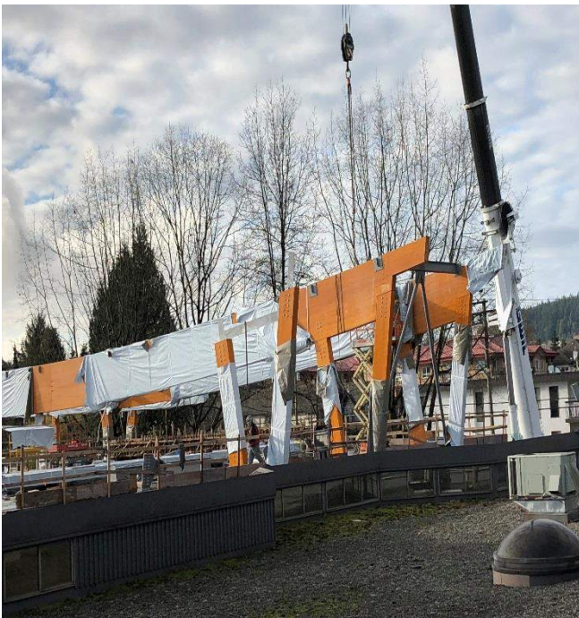
Phase C Glulam structural bracing installation looking southwest
