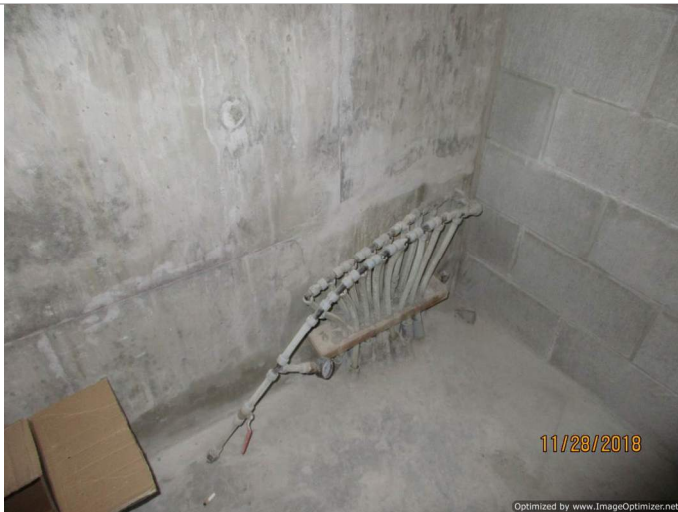
Photo 7: Radiant manifold location by door swing Of changeroom 8
