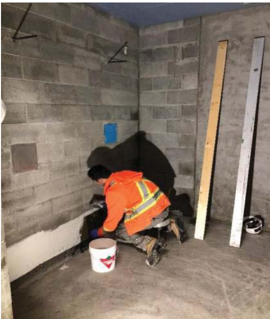
Phase 1A Change Room concrete preparation for tiling
