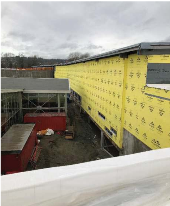
Densglass Public Corridor 1B118 south elevation
