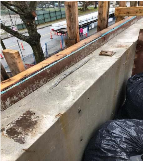
Phase 1C Level 2 wall along GL 1C-1 rebar protruding through top of wall.
