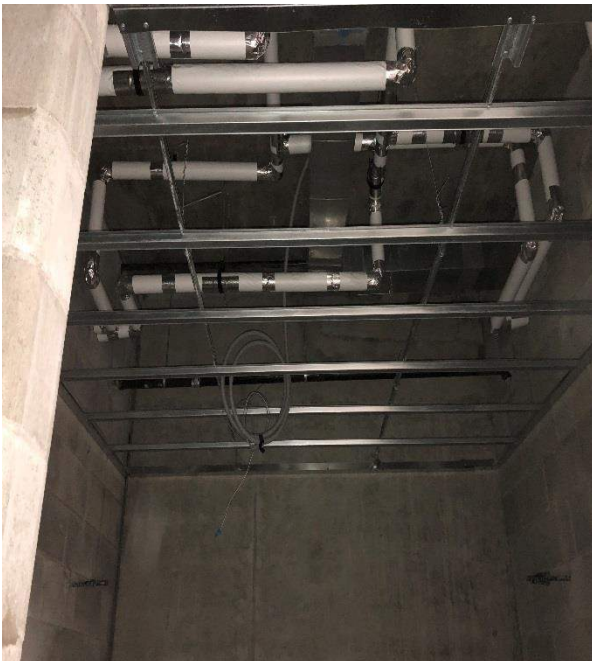
Level 1 Change Rooms ceiling framing.
