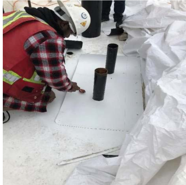
Mechanical roof membrane around penetrations.
