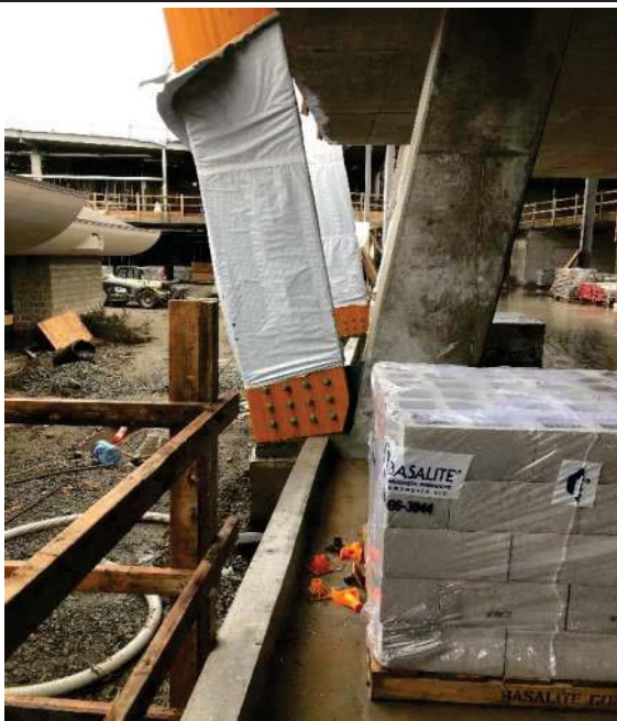
Phase 1C Level 1 curbs poured along GL 1C-A.
