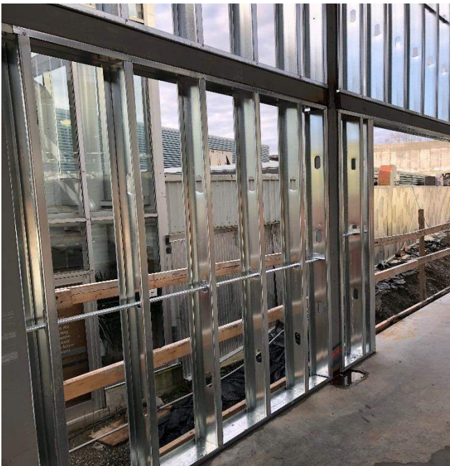
Public Corridor south wall steel stud framing
