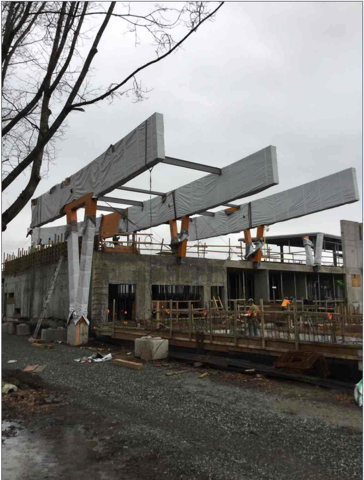
Phase 1C – Glulam installation
