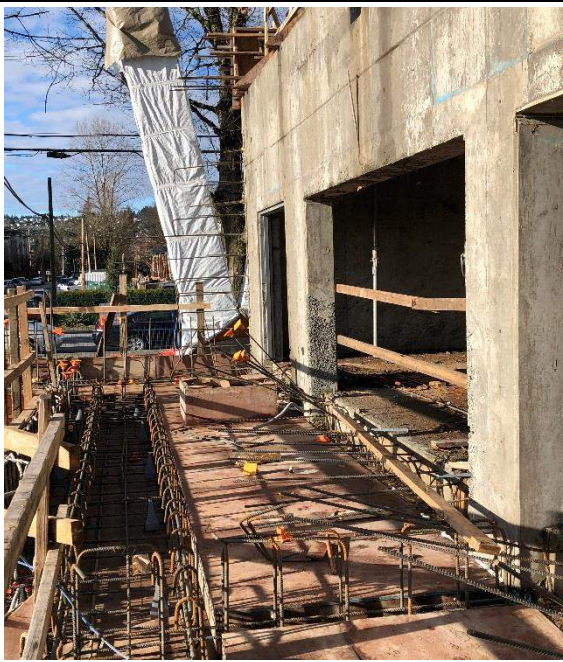
Phase 1C Level 1 Pool slab formwork.
