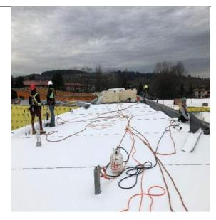
Public Corridor 1B118 roofing membrane and welding. Roof type R1
