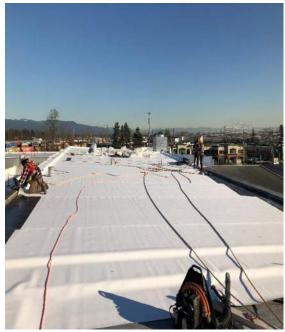
Public Corridor 1B118 roofing membrane and welding. Roof type R1.
