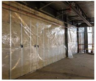
Level 2 north wall along GL 1A-H between 1A-1 & Level 2 north wall along GL 1A-H between 1A-1 & 1A-2+ AVB to be sealed. Wall type 7.
