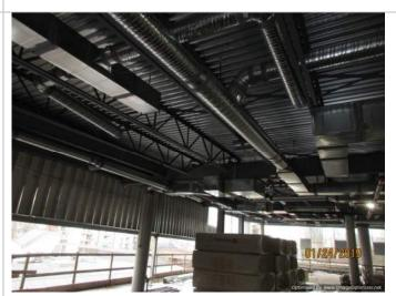
Photo 6: Ductwork in Phase 1AB (Level 2 Library)
