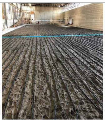
Rink 3 under rink heat piping and backfill
