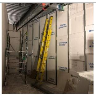
Level 2 Storage 1A216 south shaft wall firestopping to be completed. 2hr FRR
