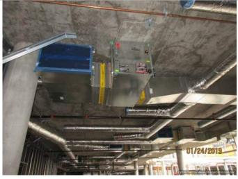
Photo 5: Heat Pump and ductwork, P-1AB Library.
