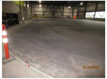
Photo 7A: Rink 2 Slab concrete topping
