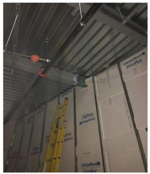
Level 2 Storage 1A216 south shaft wall and steel stud north wall. 2hr FRR
