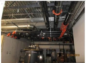
Photo 13: Hydronic Piping and duct mains suspended from roof/ceiling structure above in second floor Mech Rm.
