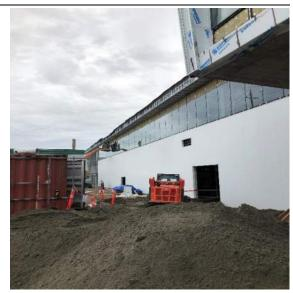
Rink 3 north face Curtain Wall glazing and spandrel panels between GL 1B-9 & 1B-11-looking southeast.
