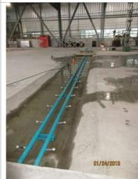
Photo 7B: Rink 3 Heating Main on depressed slab
