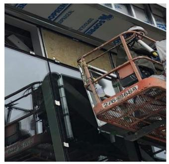
Rink 3 north face Curtain Wall glazing and spandrel panels between GL 1B-9 & 1B-11-.
