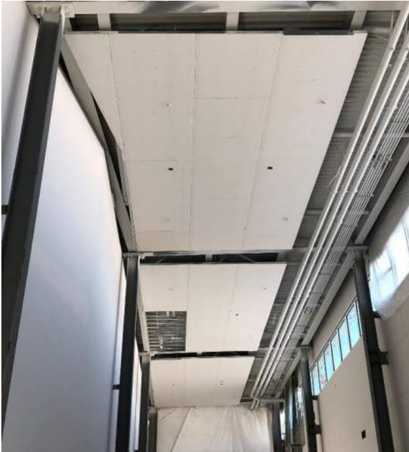
Public Corridor ceiling GWB installation
