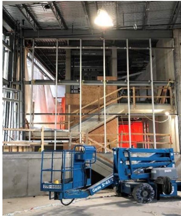
Rink 3 mullion framing at GL 1B-4 between 1B-E & F
