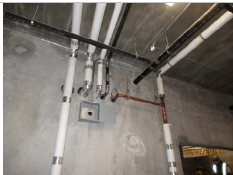
Photo #8: Water Line to Refrigeration
