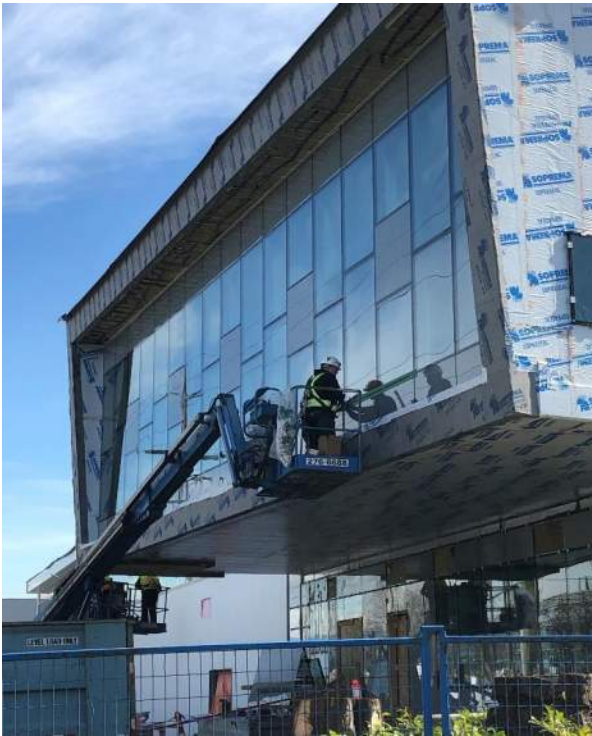
Library north elevation glazing sealing.
