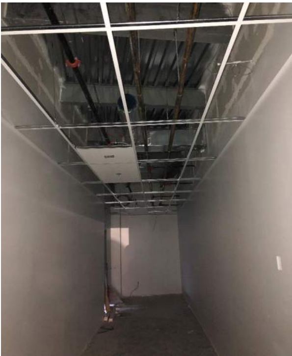
Corridor 1A213 T-Bar ceiling framing looking east
