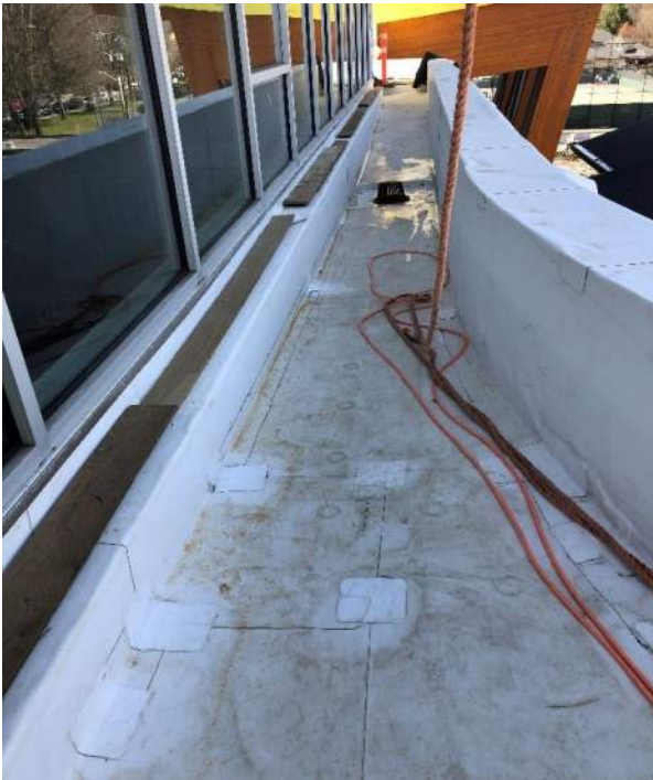
Roof Type R1 membrane repair at GL 1B-1 & 1B-F
