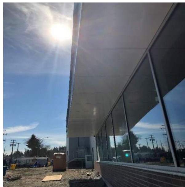
Rink 2 East elevation canopy soffit ACM Panels
