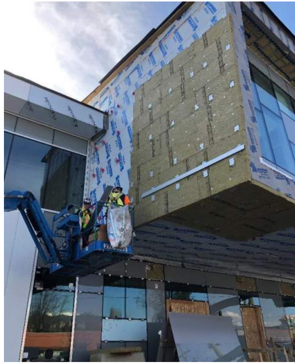
Library east elevation along GL 1B-4, AVB, insulation and thermal clips. Wall Type 4
