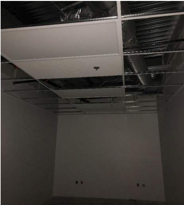
Equipment Storage 1A214 T-Bar ceiling framing and sprinklers
