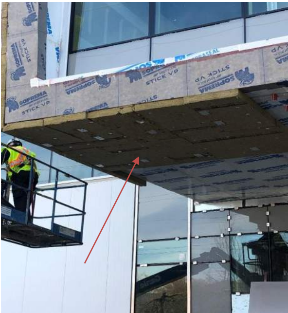
Library north elevation soffit, AVB, insulation and thermal clips. Wall Type 4a.
