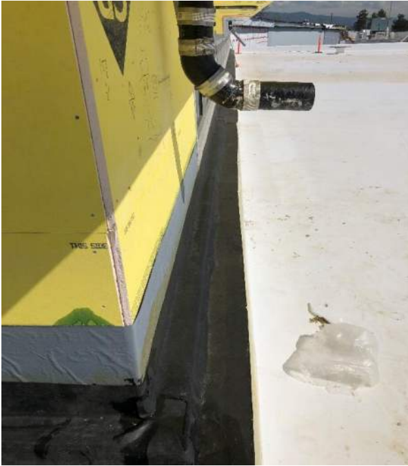
Phase 1C Expansion Joint along 1C-E at Administration roof level looking east.
