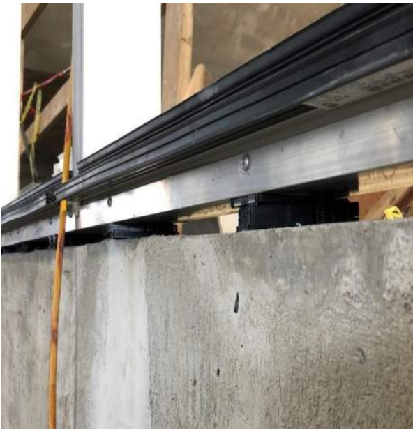
Rink 3 mullion framing/shimming at GL 1B-4 between 1B-E & F
