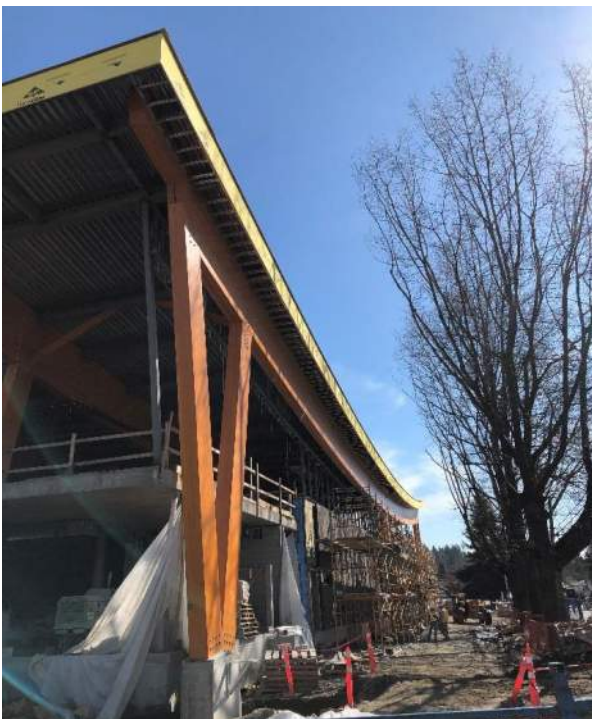
Phase 1C North and West Elevations parapet sheathing.
