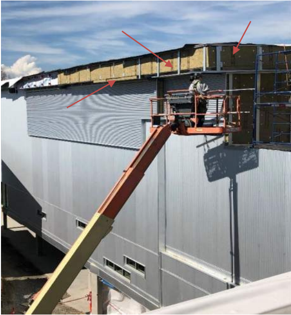
Public Corridor south elevation at GL1B-14 & 1B-F insulation at u/s and front face of parapet. Wall Type 5.
