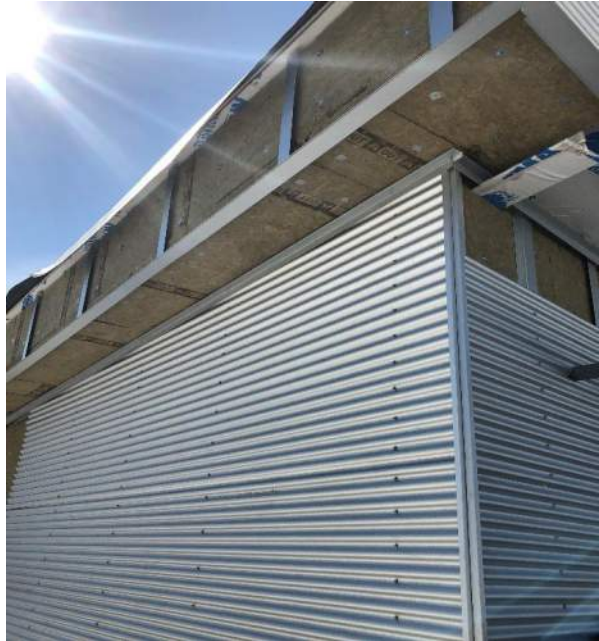
Public Corridor east & north elevation at GL1B-14 & 1B-F insulation at u/s and front face of parapet. Wall Type 5.
