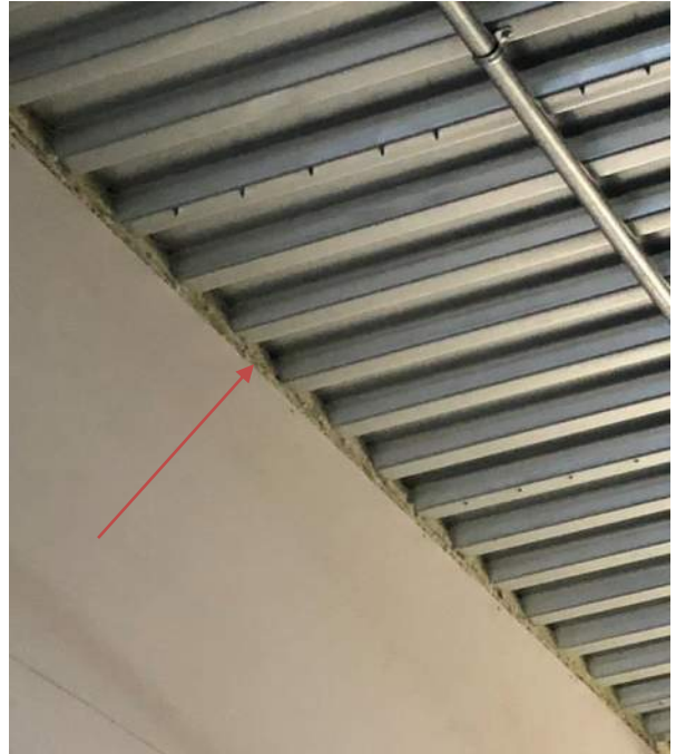
Phase 1C Level 2 GL 1C-11+, Circulation 1C200 firestopping (mineral wool)
