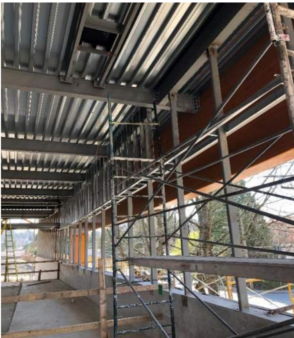
Phase 1C roof soffit framing along GL 1C-1+
