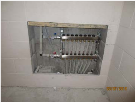
Photo #3: Radiant Floor Manifold
