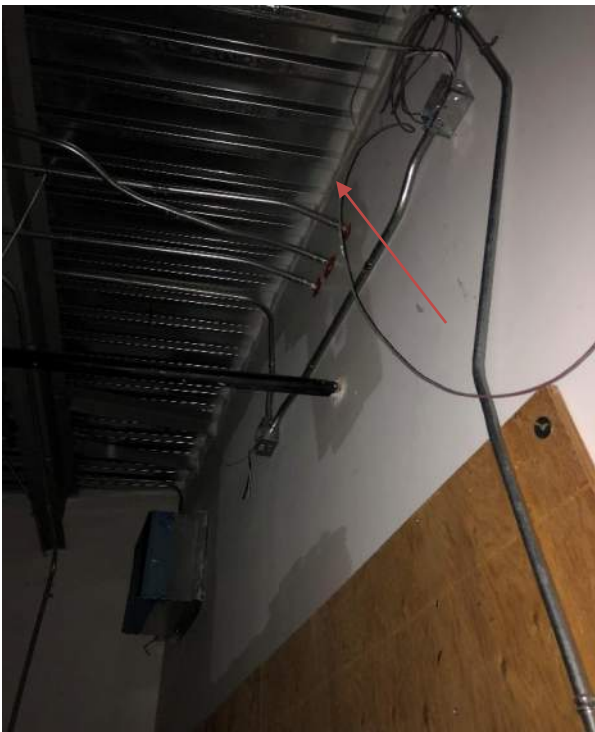
Electrical Room 1A215 east wall firestopping
