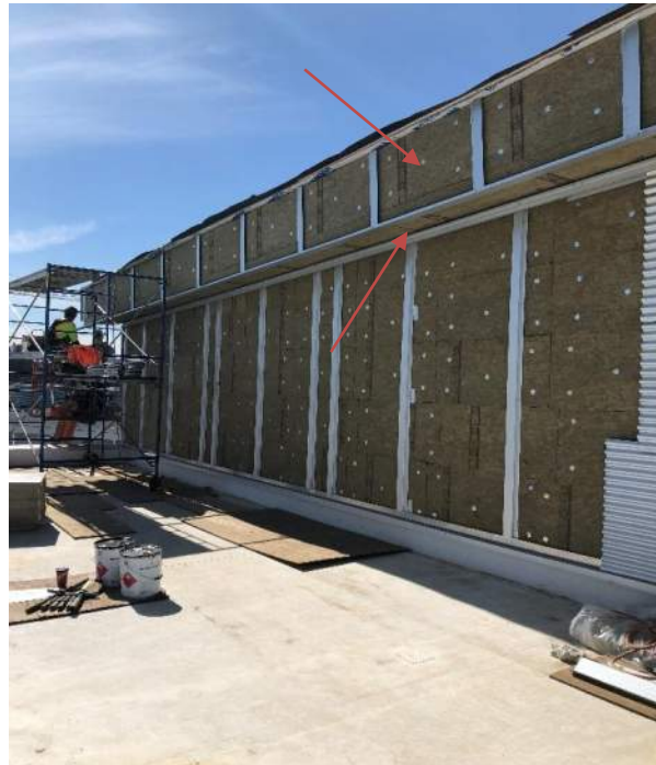
Public Corridor along GL1B-14 between 1B-F & 1A-H insulation at u/s and front face of parapet. Wall Type 5.
