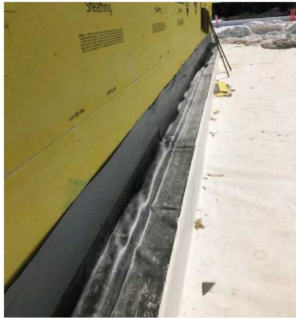
Phase 1C Expansion Joint along GL 1C-7 west end of corridor roof level looking south.
