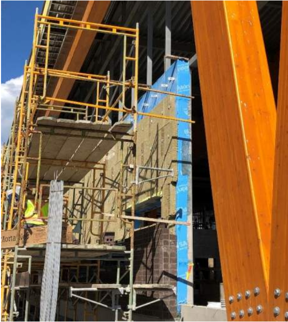
Phase 1C west elevation along Gridline 1C-1 between 1C-C & 1C-P, AVB, insulation and thermal clips. Wall Type W1
