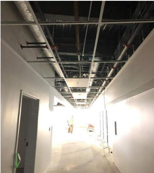
Corridor 1A213 T-Bar ceiling framing looking west
