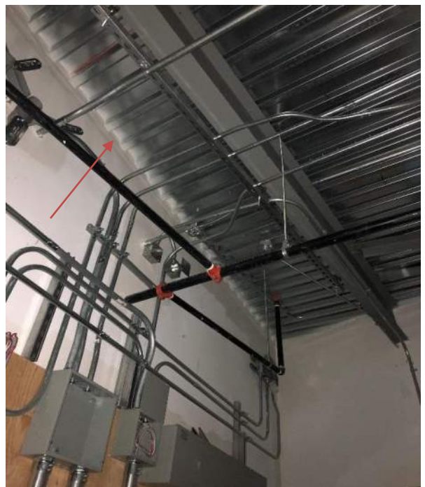
Electrical Room 1A215 west wall firestopping
