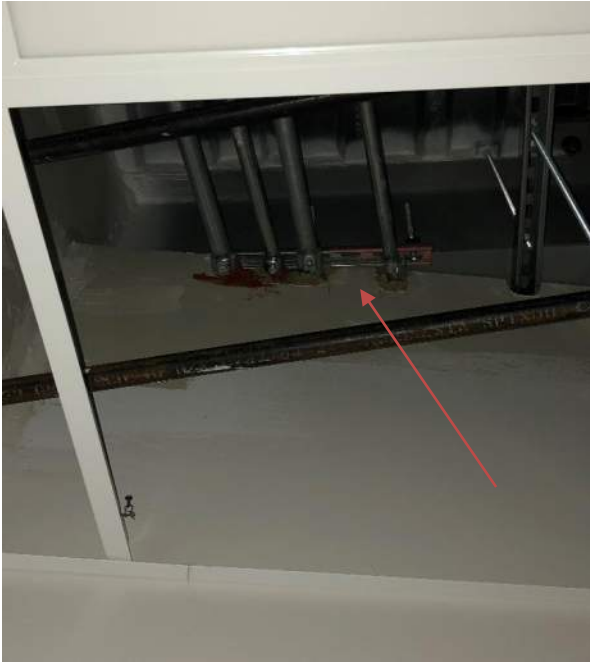
Equipment Storage 1A214 east wall electrical firestopping to be completed.
