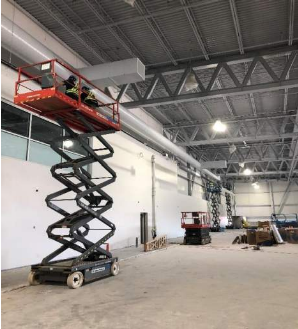
Rink 2 Radiant heater lines at west side
