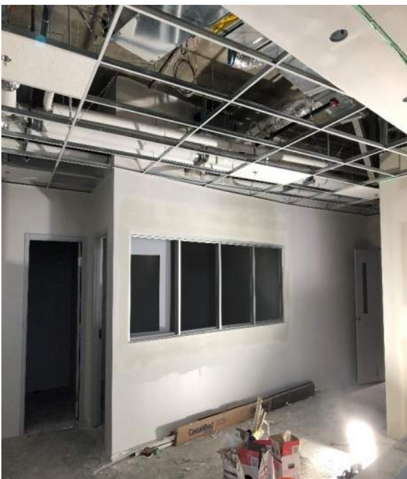
Service Point 1A125 T-Bar ceiling framing.
