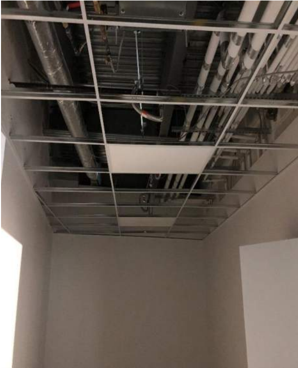
Concession Storage 1A212 T-Bar ceiling framing and sprinklers
