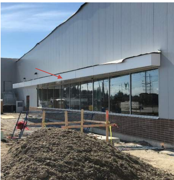
Rink 2 East elevation canopy east face ACM Panels
