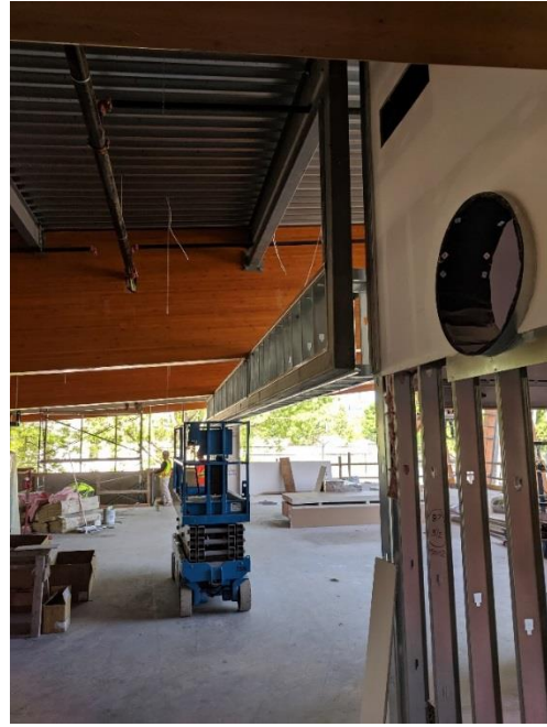
Level 2 Fitness room 1C230 bulkhead, in progress.
