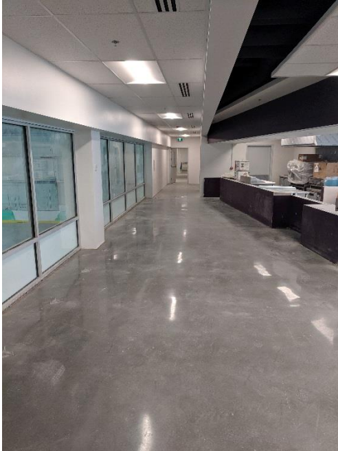
Concession 1A211 Polished Concrete Floor.
