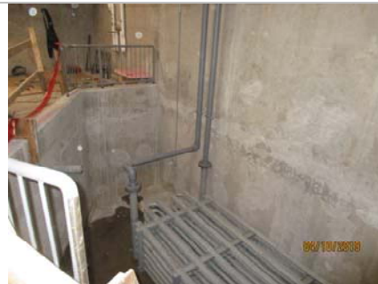
Photo #6: Ice Melt Pit Coil Piping
