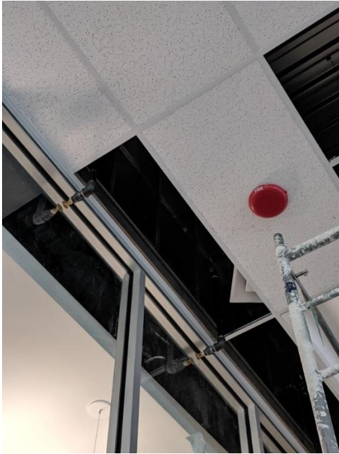
Stair 4 - 2 hour rated gypsum wall to be installed above glazing.
