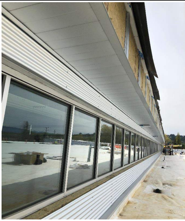
Public Corridor north elevation roof eave soffit insulation and metal panels. Wall Type W5
