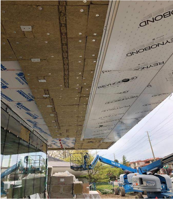
North face Library soffit. Wall Type W4a
