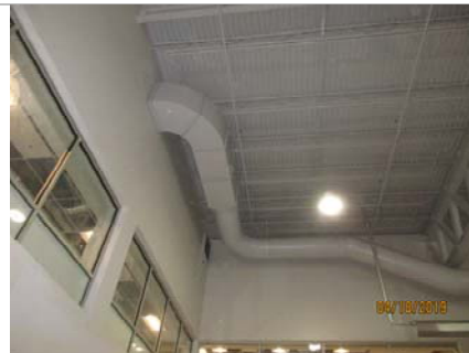
Photo #8: Supply Air ducting
