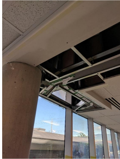
Library Level 1 sliding door #1B150B seal bulkhead to mullion.
