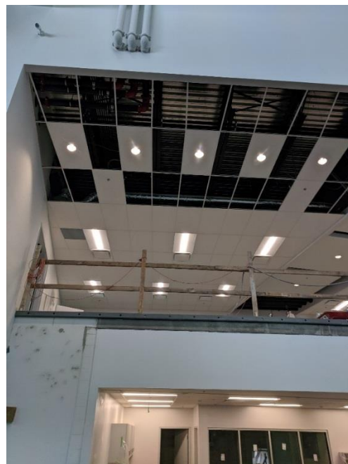
Level 2 acoustical ceiling in progress.
