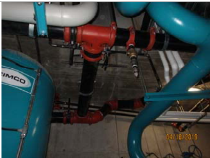
Photo #5: Thermal Equalizer Tank Piping
