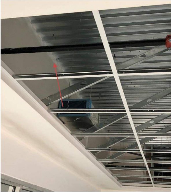
Level 2 Administration smoke seal at top of wall/deck interphase.
