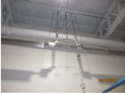
Photo #1: Rink #2 Radiant Heaters
