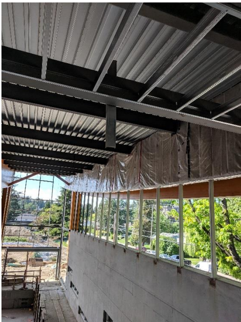
Pool west elevation bulkhead AVB.
