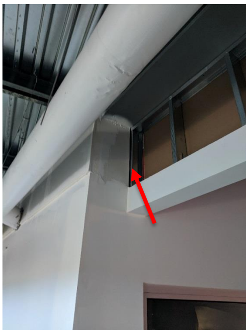
P1C Level 2 admin bridge to fitness, Gypsum board to be sealed around bulkhead.
