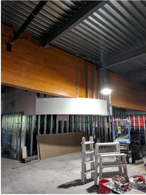
Level 2 Fitness office 1C233 bulkhead, in progress.
