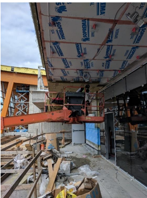
AVB and thermal clips outside of 1C113.
