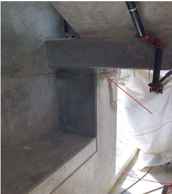
Stair 1 south wall epoxy injection remedial work completed.
