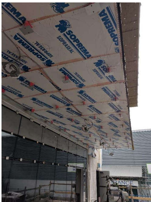
AVB and thermal clips outside of 1C113.
