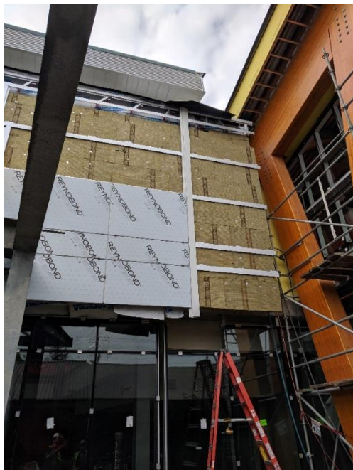
Main Entry North elevation Metal Panels in progress, insulation and expansion joint cover Wall Type W4
