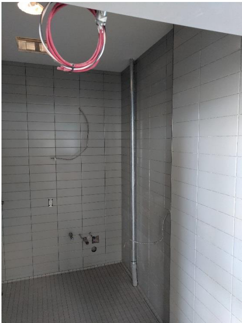
Washroom 1B262 Conduit to be covered, instruction to follow.
