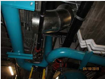
Photo #7: Refrigeration Room Exhaust
