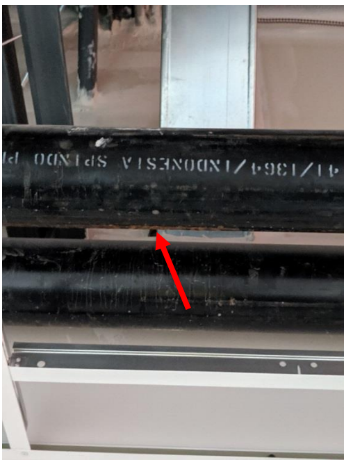
Corridor 1C200 steel stud brace firestopping to be installed at north wall.
