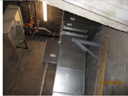
Photo #4: Refrigeration Room Air Intake
