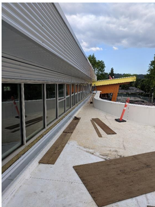
Public Corridor North side cladding and prefinished metal soffit.
