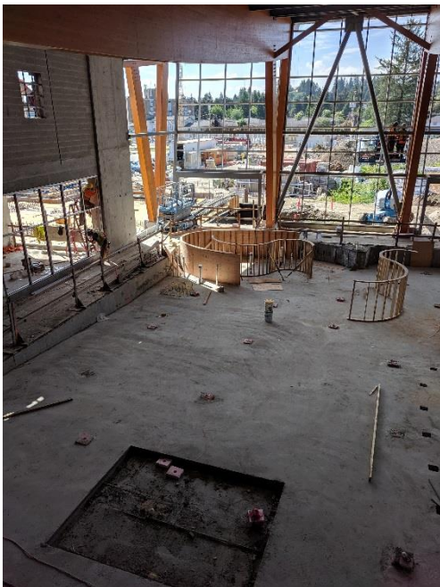
Pool slab and lazy river formwork, in progress.
