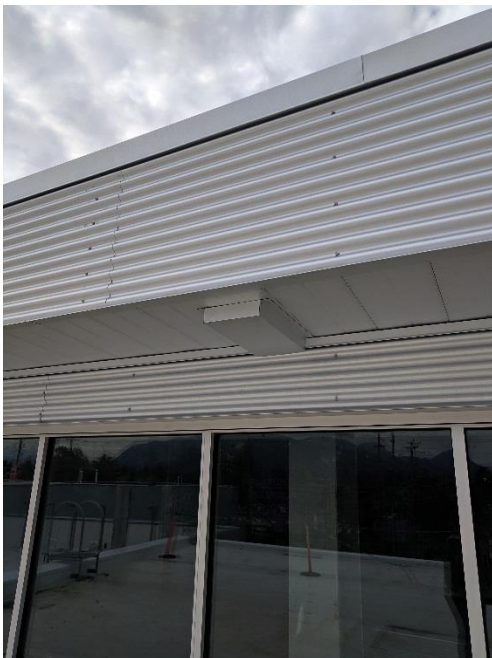
Public Corridor North Side – Prefinished metal cover at prefinished metal soffit.
