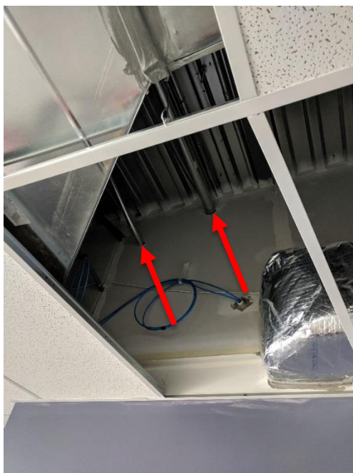
Room 1C217 Conduit firestopping to be installed at west wall.
