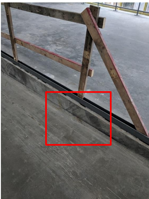
Nail protruding from concrete near top, south side of ramp in public corridor 1B118.
