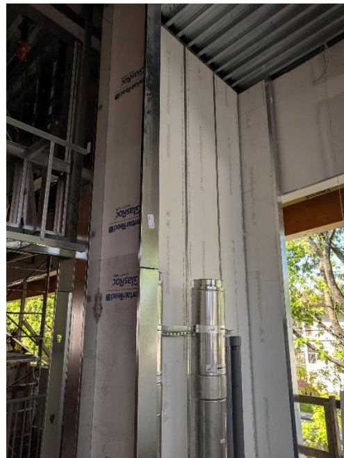
P1C Stair 3 north wall shaft liner and ducts, in progress.
