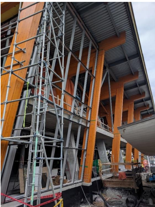
P1C North Elevation mullion installation, installation in progress.
