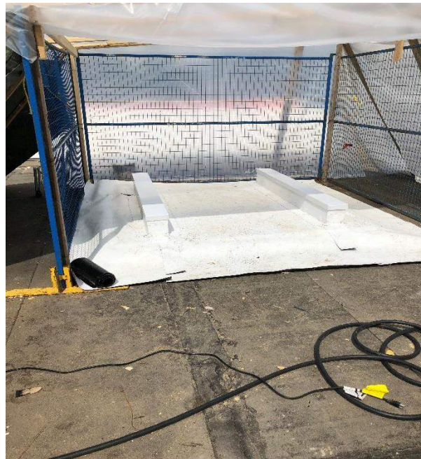
Change Room roofing membrane at mechanical unit curb
