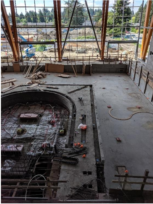
Pool slab and hot tub plumbing and formwork, in progress.
