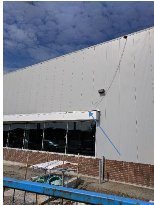
Rink 2 east canopy pre-finished cap flashing work in progress.
