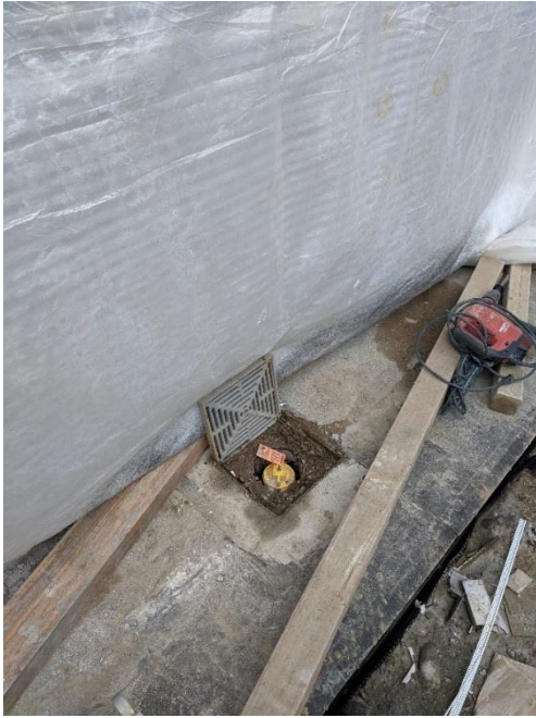
Exterior of Main Entry floor drain.
