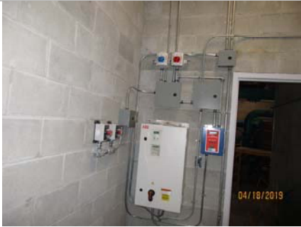
Photo #3: Ammonia Detector/Lights/Switches
