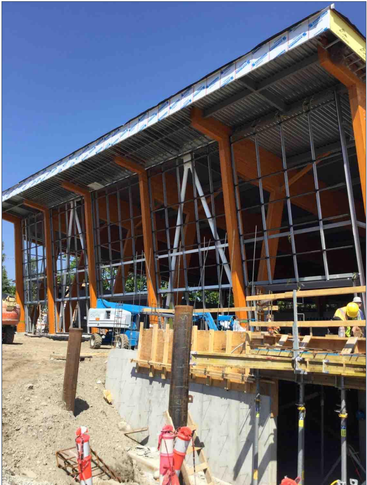
Phase 1C – South elevation glazing frame
