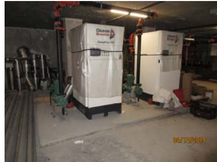
Photo #12: Phase 1C Boilers
