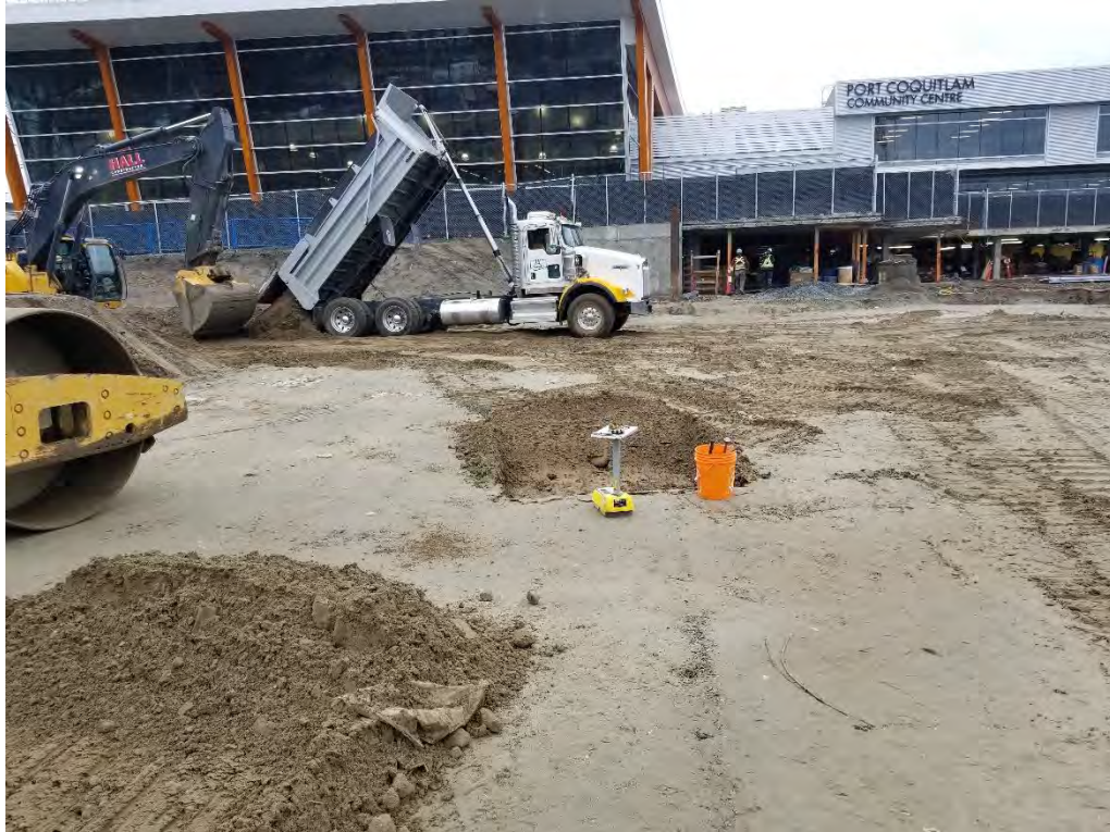
Photo 5 – Fill placement for the access ramp (Item 5). [photo taken by JAL and dated 20191118]
