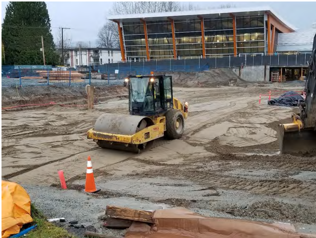
Photo 4 – Compaction of river sand fill at south end of excavation (Item 4). [photo taken by JAL and dated 20191118]
