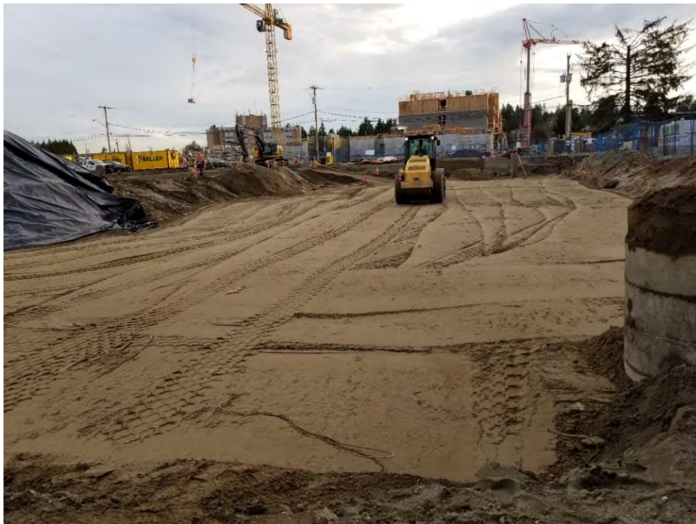
Photo 6 – Recompacting of third lift for the second time. [photo taken by JAL and dated 20191114]
