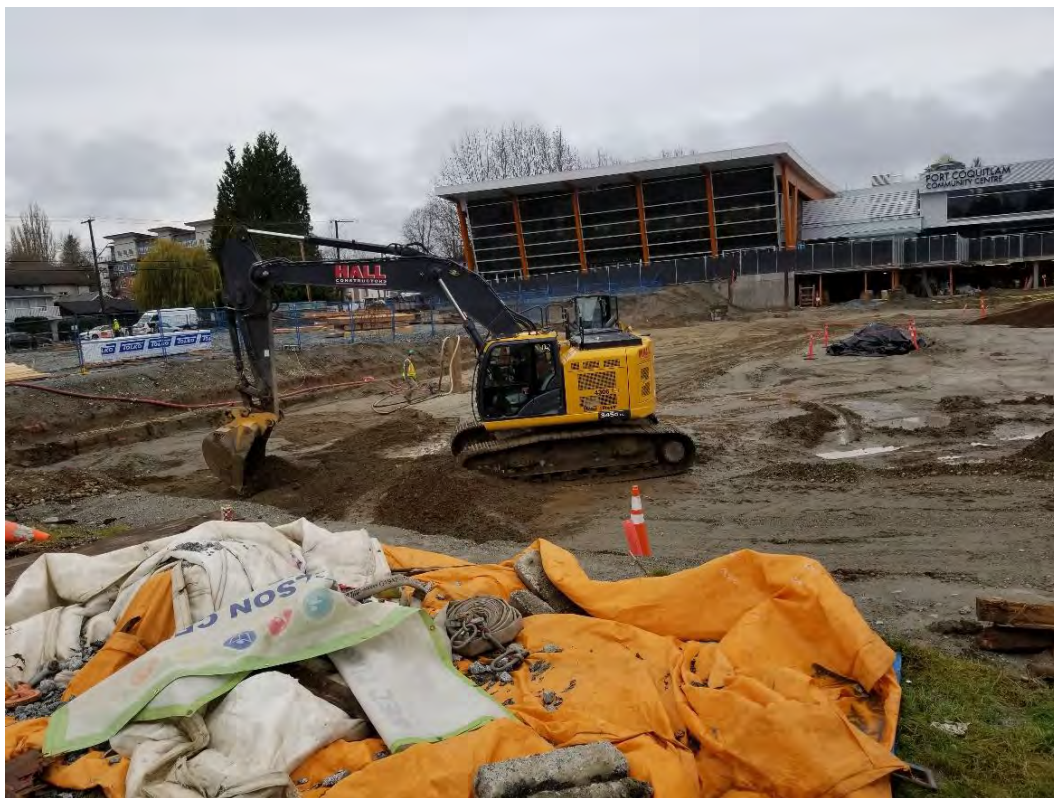
Photo 2 – Removal of standing water and saturated material along south end of excavation (Item 4). [photo taken by JAL and dated 20191118]
