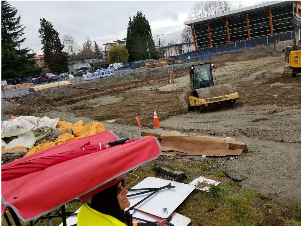
Photo 3 – Compaction of the disturbed surface prior to fill placement (Item 4). [photo taken by JAL and dated 20191118]
