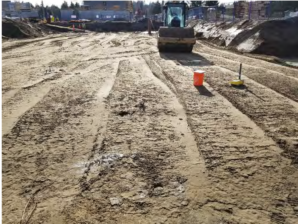
Photo 3 – Second lift placed across the approved subgrade area (Item 6). The base of the entire is now flat (Item 7). [photo taken by JAL and dated 20191114]
