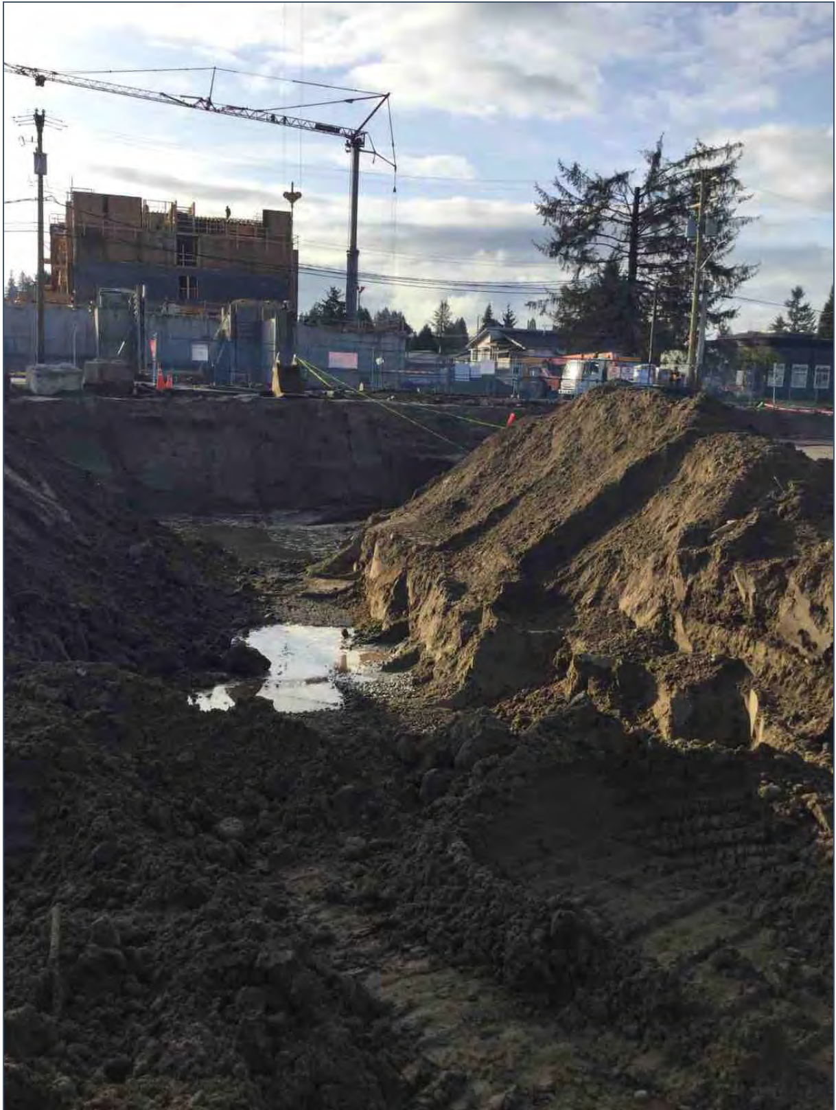
Phase 2 – Bulk Excavation
