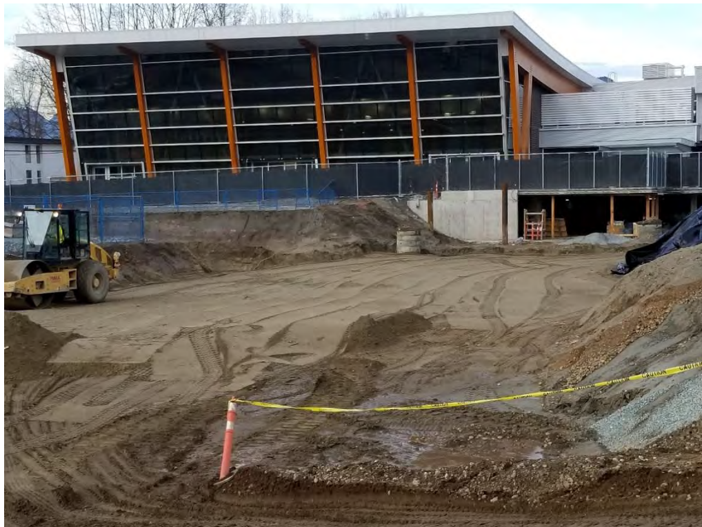
Photo 4 – During compaction of the last lift of fill (Item 9). The lift extended from the north of the excavation up to the well point near the southwest edge of the of the excavation. [photo taken by JAL and dated 20191114]
