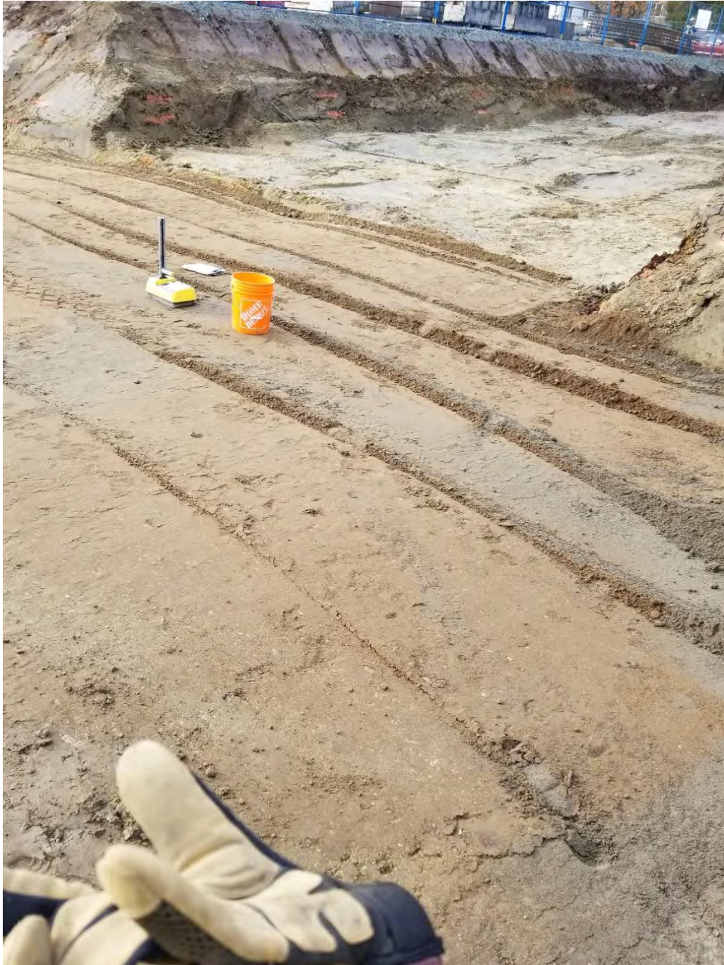
Photo 2 – A lift of Sand and Gravel placed over the west portion of the approved subgrade area. The lift varied in thickness to level out the sloping subgrade (Item 5). [photo taken by JAL and dated 20191114]
