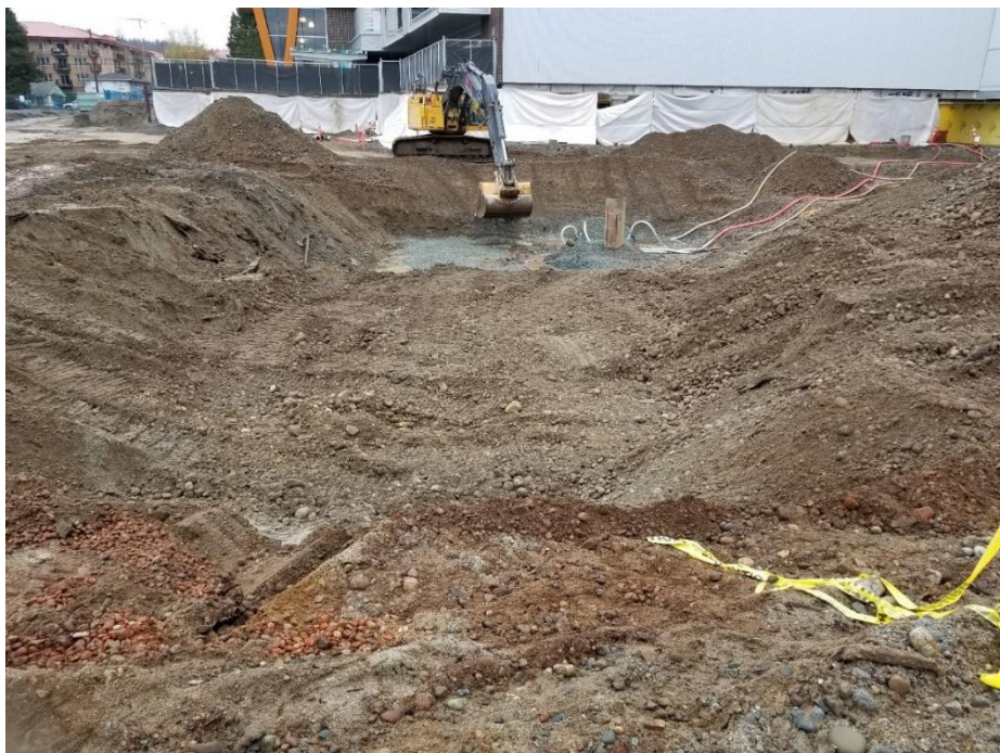
Photo 2 – Looking west. Locally placing 19 mm minus clear crush at the base of the excavation (Item 3). [photo taken by JAL and dated 20191203]
