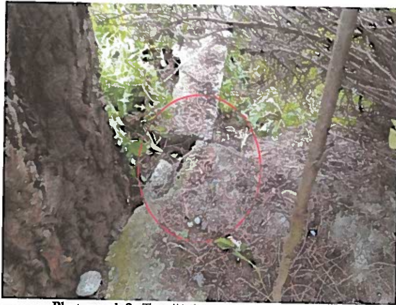
Photograph 2: Tree #1 damage to the retaining wall.
