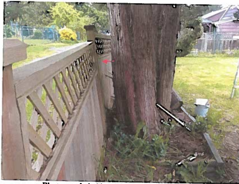
Photograph 4: Tree #2 pushing out the fence.
