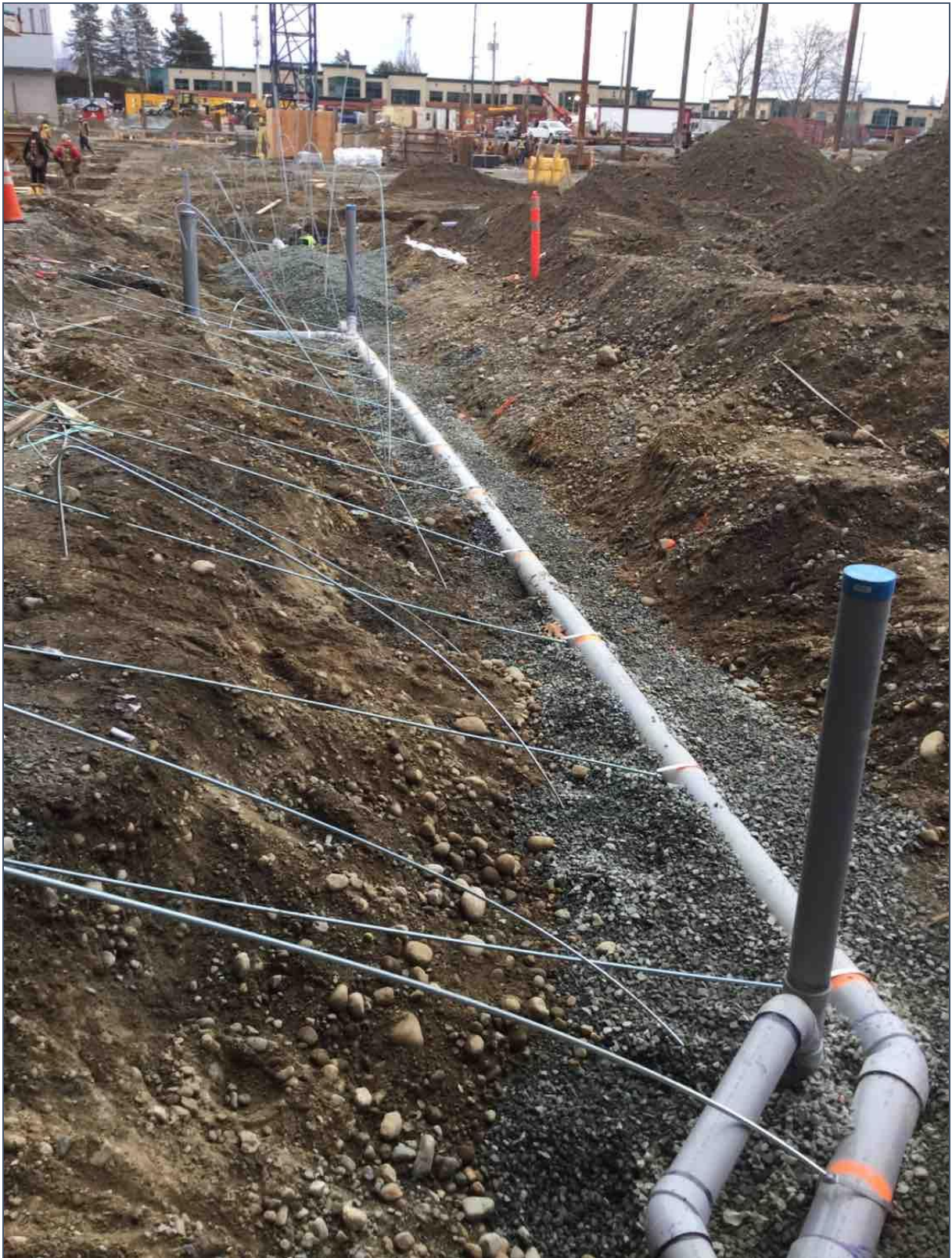
Phase 2 – Under slab drainage
