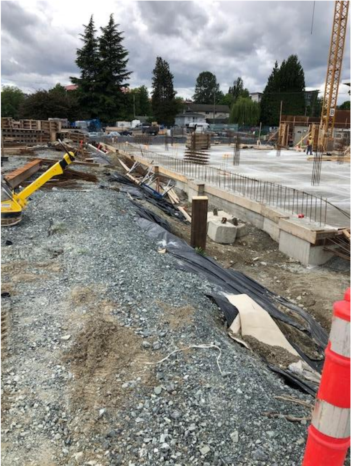
Phase 2B – Parkade walls formwork preparation
