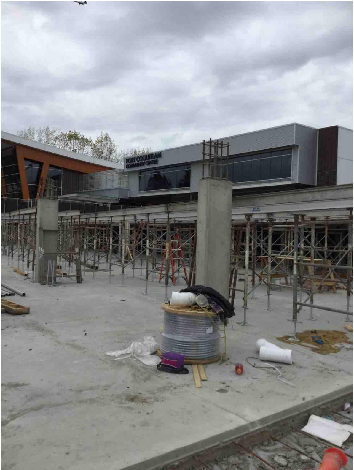
Phase 2B – Parkade suspended slab falsework preparation
