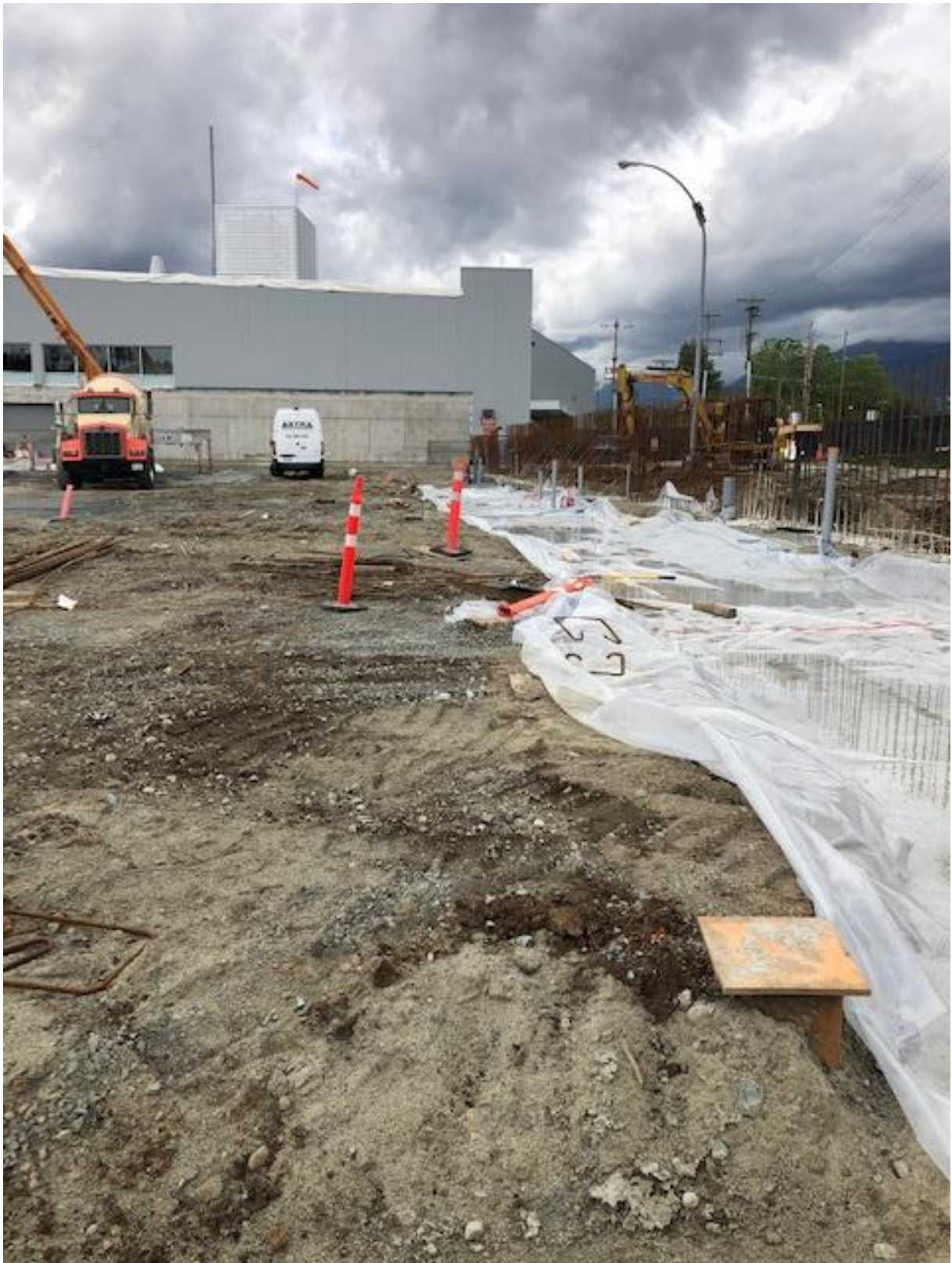
Phase 2A – Rink refrigeration pipework & slab preparation
