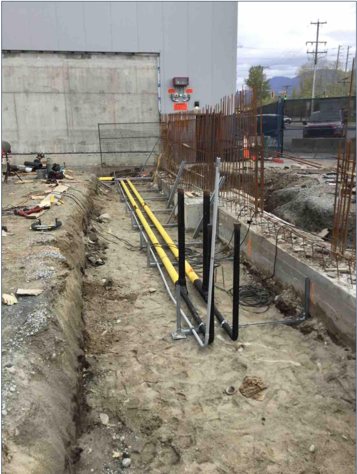
Phase 2A – Rink refrigeration pipework
