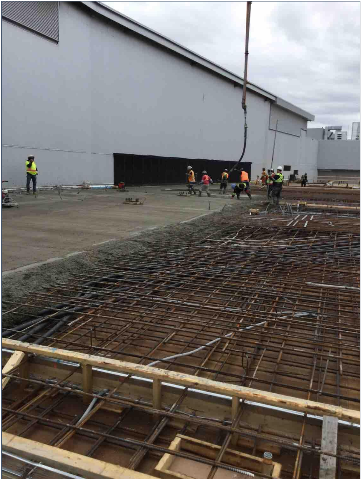
Phase 2C – Parkade suspended slab concrete placement
