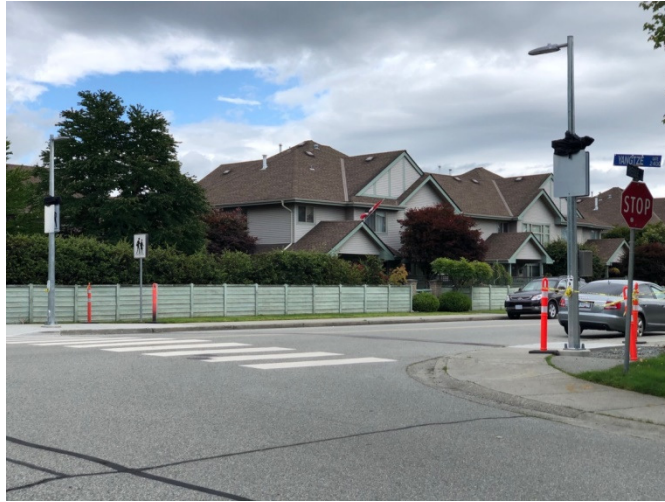
RRFB at Riverside Drive and Yangtze Place
