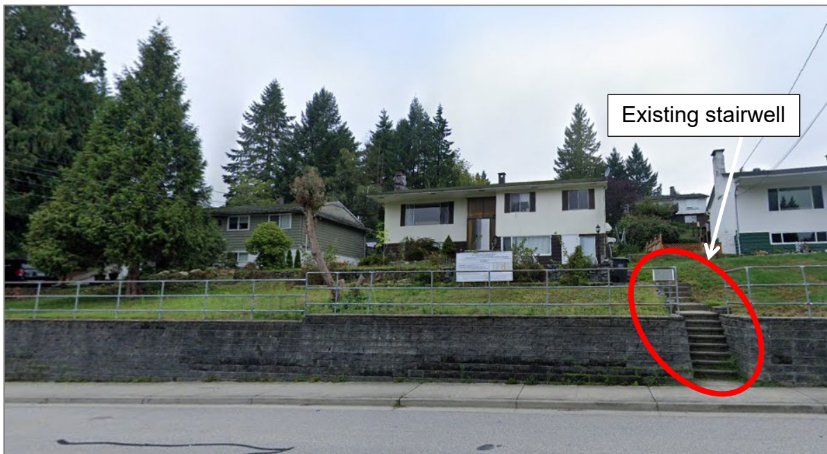
Street Front Retaining Wall
