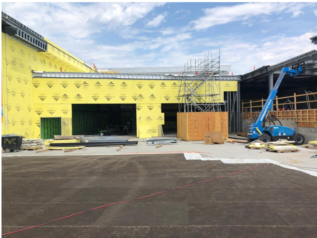
Phase 2C – Childminding envelope progress
