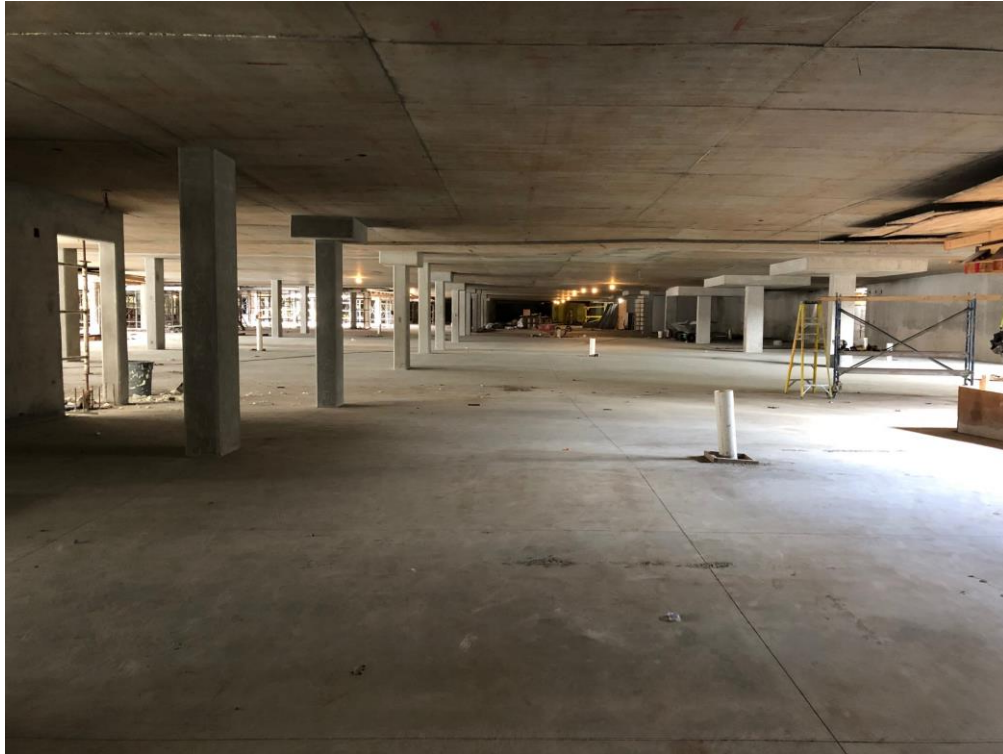
Phase 2B – Parkade underpropping removed
