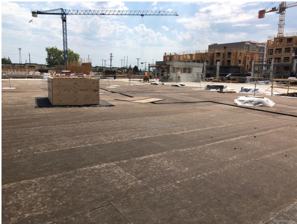
Phase 2B – West side of parkade traffic membrane progress
