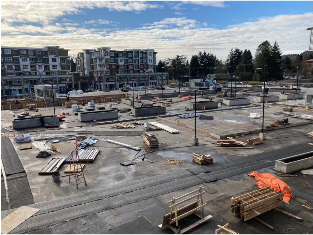
Phase 2B – South plaza finishing ongoing
