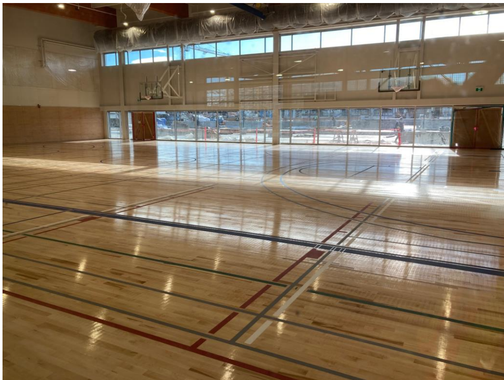
Phase 2C – Gymnasium progress
