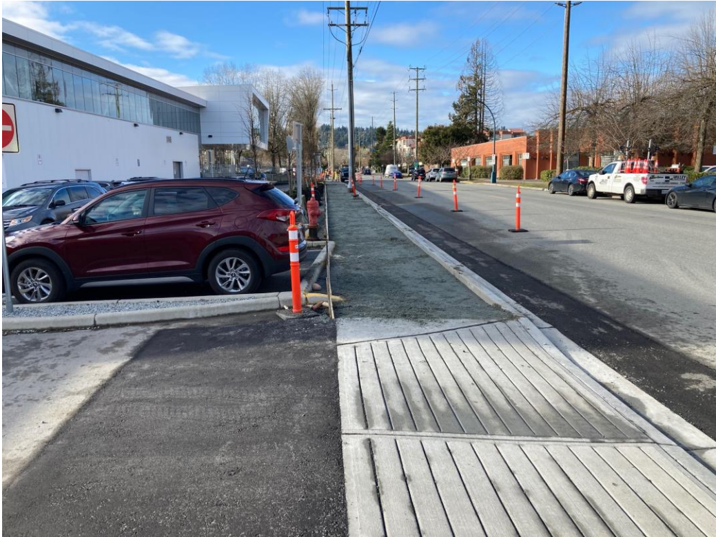
Offsite paving commenced
