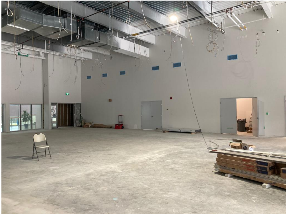
Phase 2C – Large MP Room progress
