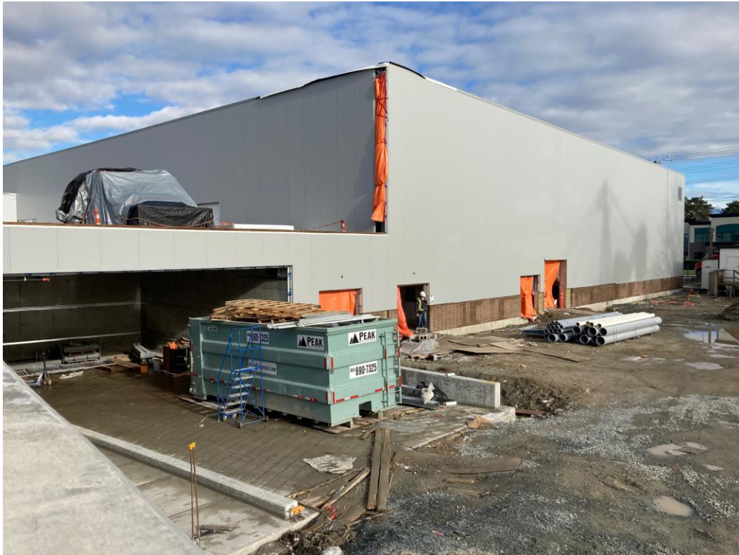
Phase 2A – Rink envelope progress
