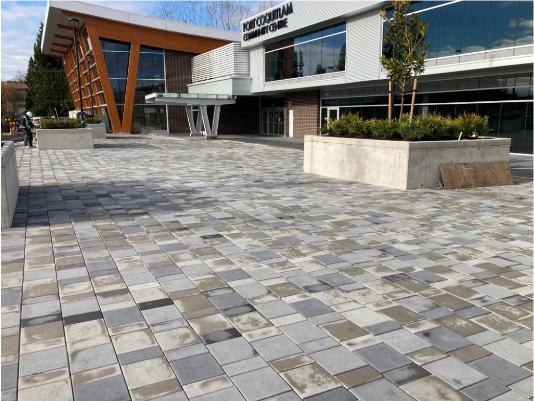
Phase 2B – South plaza paving ongoing
