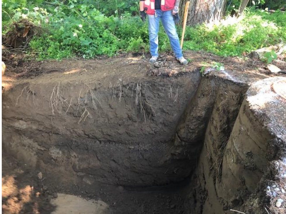
Example #5: Shows excavation work 2.8m from the tree, no structural roots were exposed.
