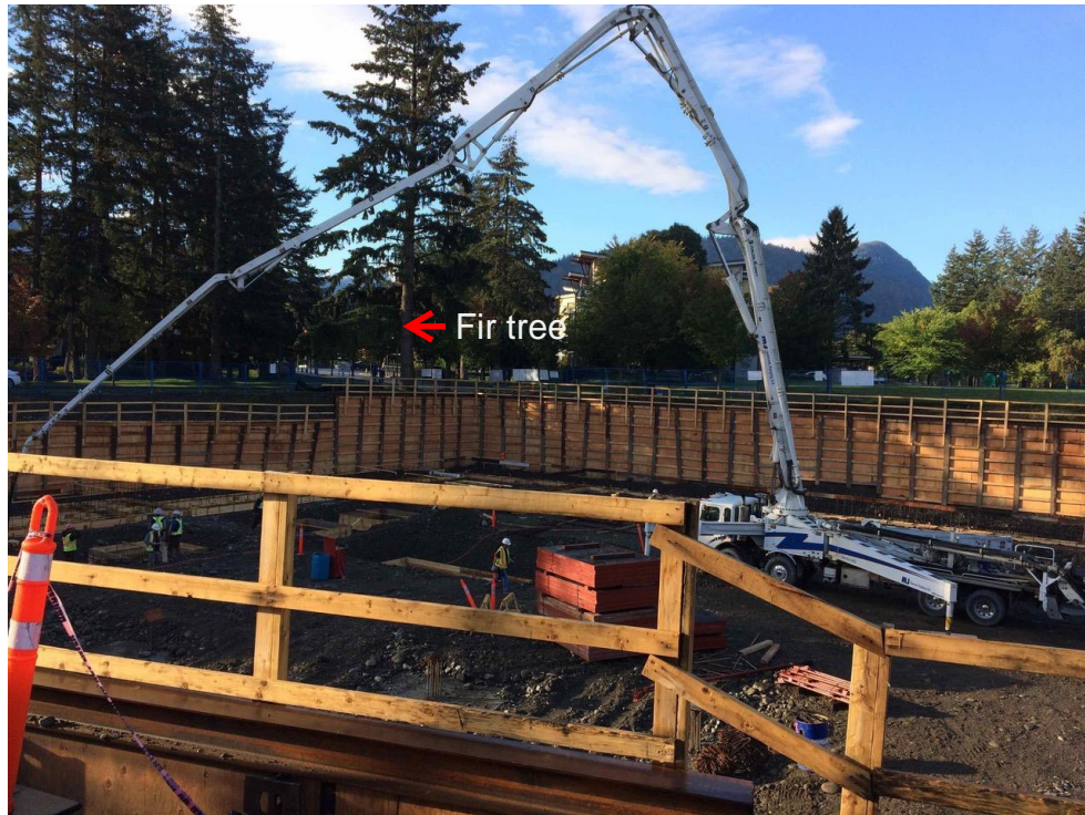
Example #3: This is an example of where piling were installed 2 meters from the base of a fir tree.
