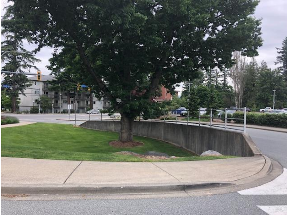
Example #4: A retaining was installed 2 meters from the Oak tree in this photograph. Approximately 10 years later the tree still shows no sign of decline.
