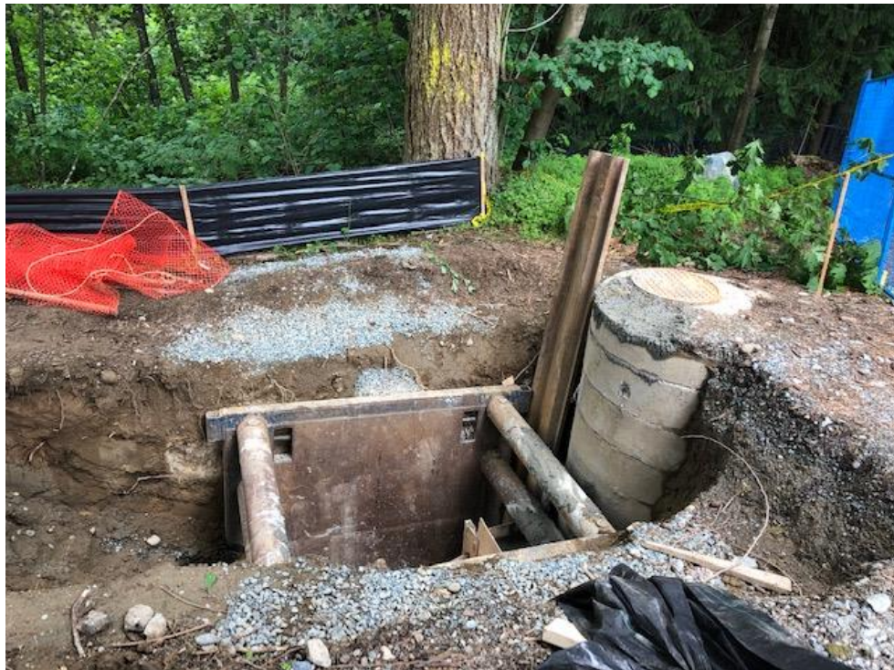
Example #5: View of shoring to support soil around the root system during excavation.
