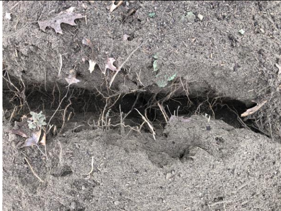
Photo 11: Only small feeding roots were discovered, no structural roots in 3 trenches.
