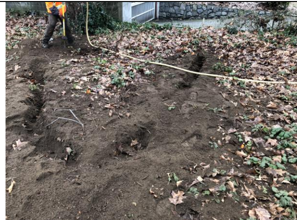
Photo 10: 3 trenches in total were made
