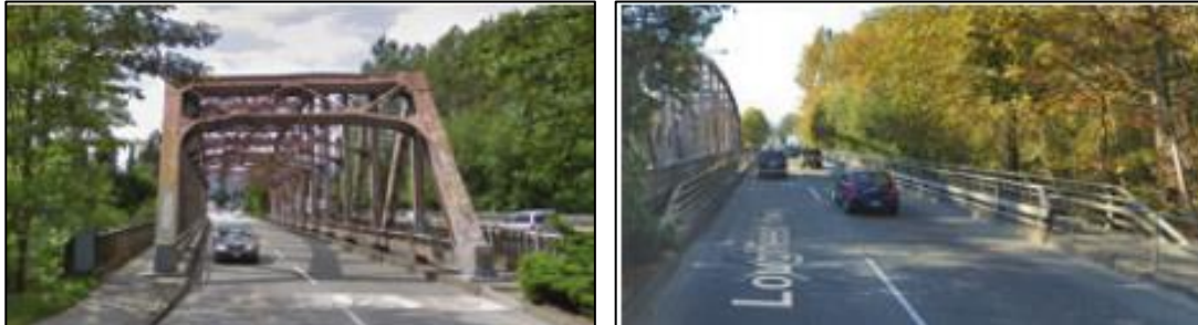
Eastbound Steel Truss Bridge (left) & Westbound Concrete Bridge (right)
