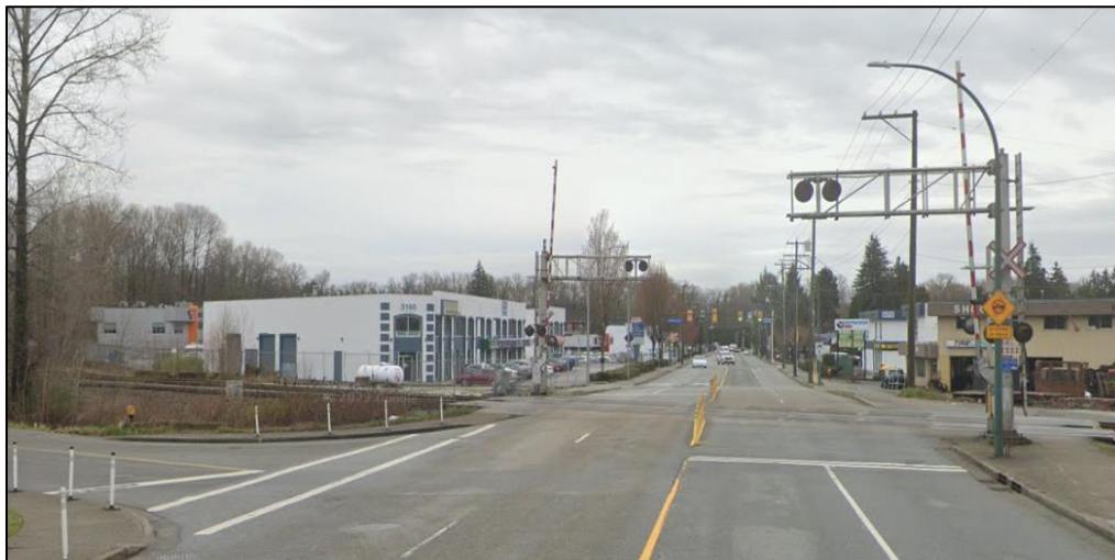
Westwood Street at Davies Avenue – Existing At-Grade Crossing
