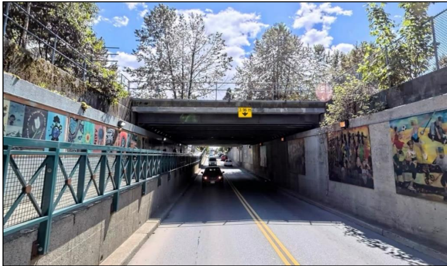
Shaughnessy Street Underpass (looking south)
