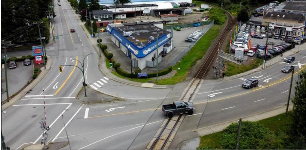
Westwood Street at Kingsway Avenue - Existing At-Grade Crossing
