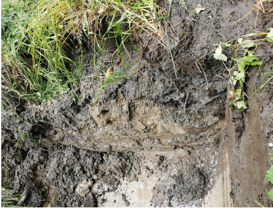
Photo 03: Test Hole Test (TH22-02) – Surficial Water Inflow
