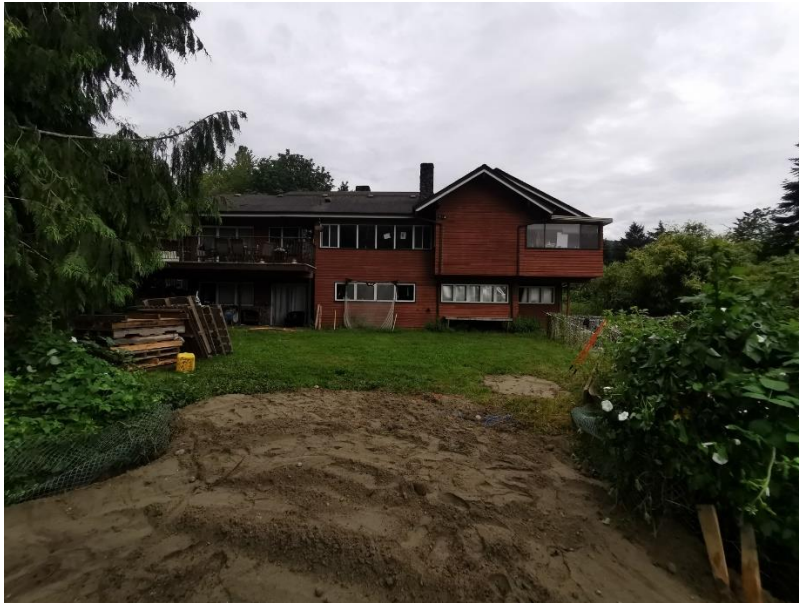
Photo 14: View of Current Building – North facing
