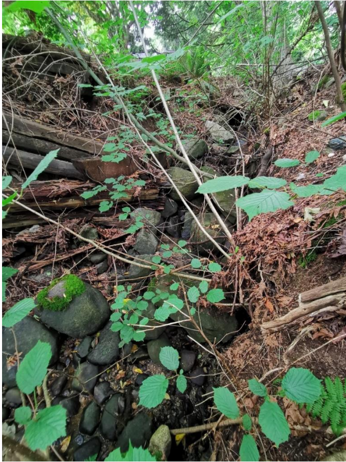
Photo 09: Upstream Ravine Area – Culvert Outlet
