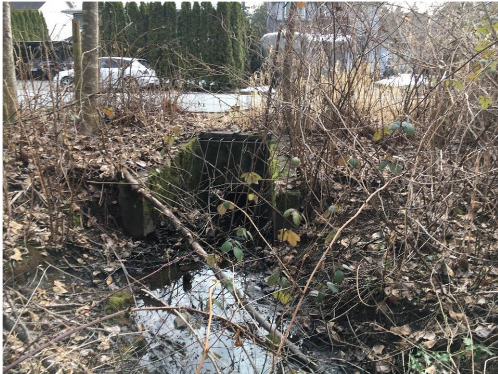
Photo 8: View of the headwall and culvert where the unnamed stream discharges into the storm sewer that crosses Lynwood Avenue.
