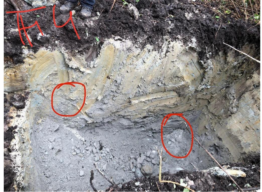
Photo 04: Test Hole Test (TH22-04) – Groundwater Seepage
