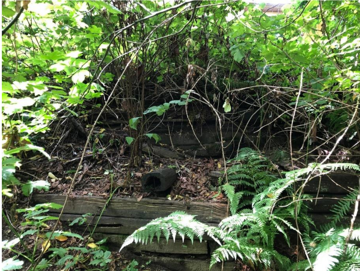
Photo 11: Upstream Ravine Area – Timber Tie Wall
