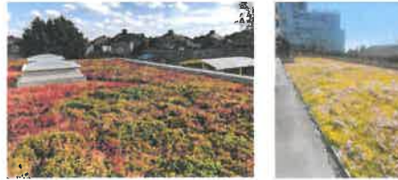
Extensive Green Roof
