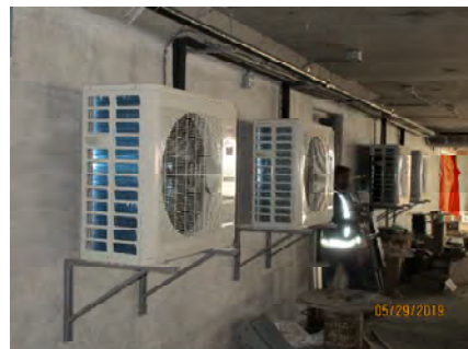
Photo #16 - Condensing Units SCU-1, 2, 3, 4
