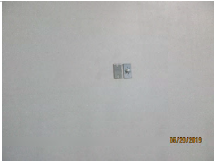
Photo #1: Arena Radiant Heater Timer
