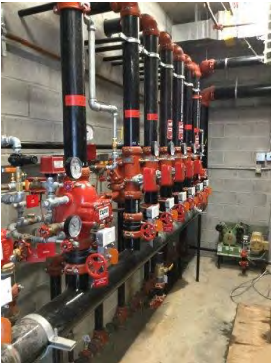
Phase 1B – Sprinkler tree ready for labelling
