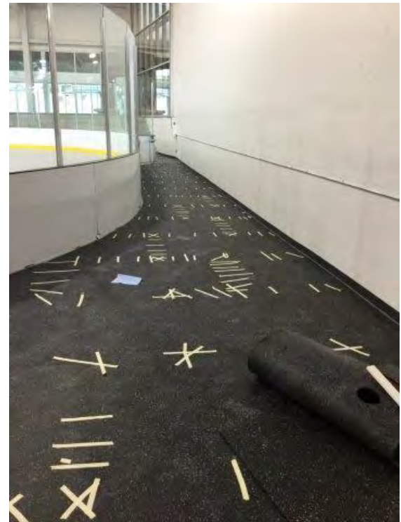
Phase 1B – Rubber skate flooring install
