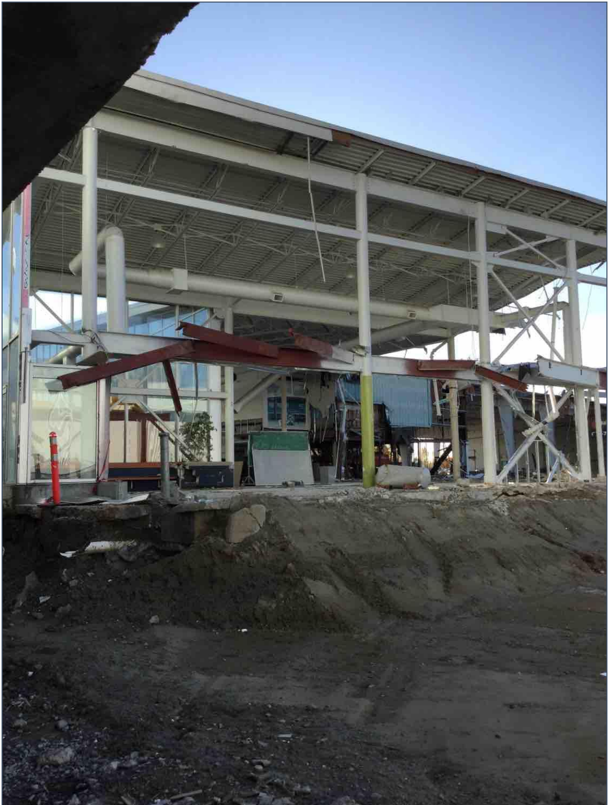
Phase 2 – Old reception demolition
