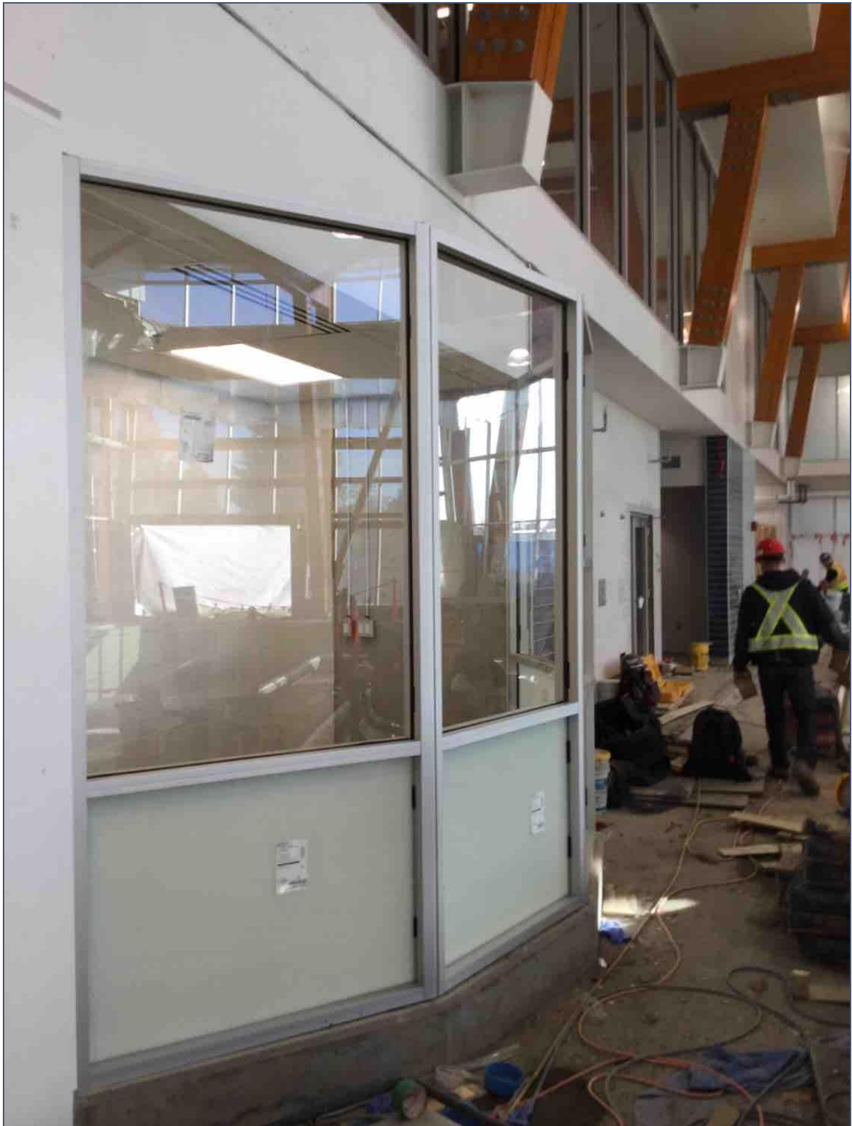
Phase 1C – Lifeguard room glazing
