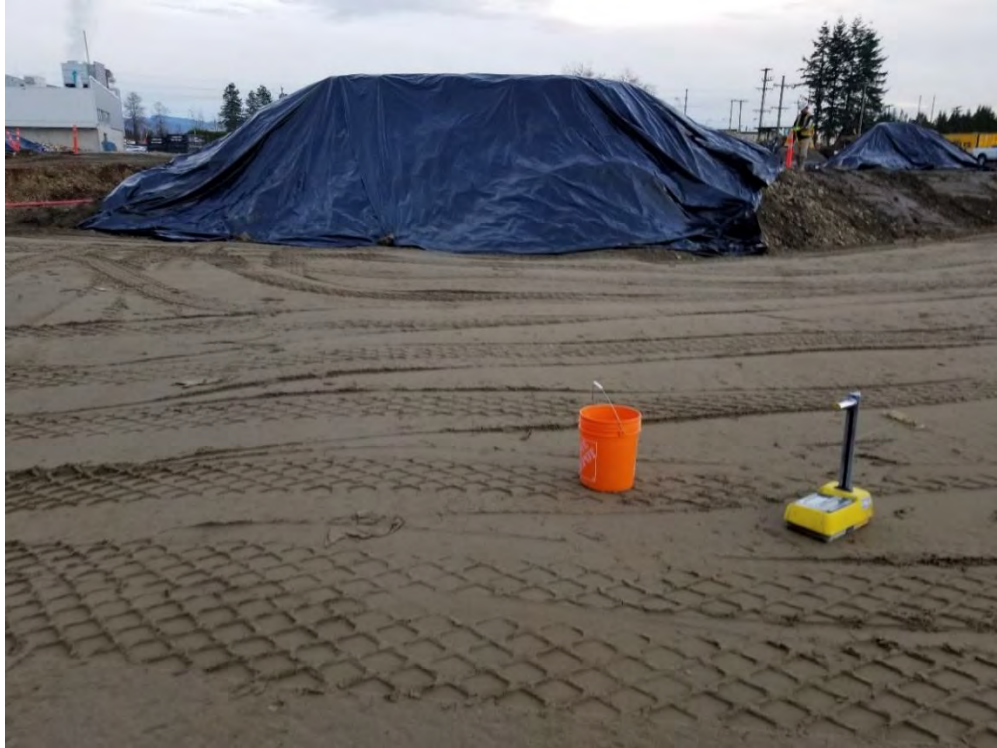
Photo 5 – Testing of third lift. [photo taken by JAL and dated 20191114]
