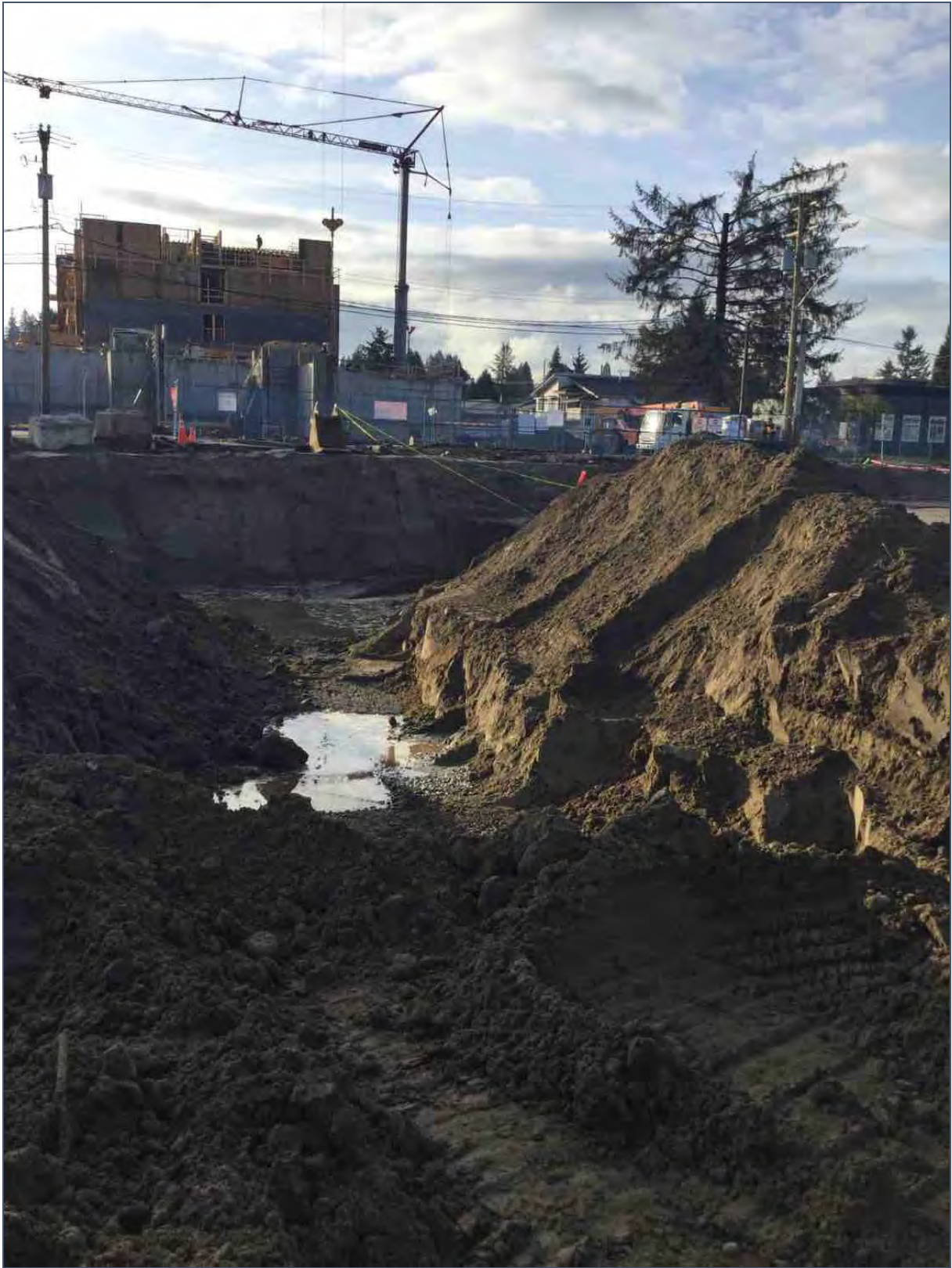
Phase 2 – Bulk Excavation
