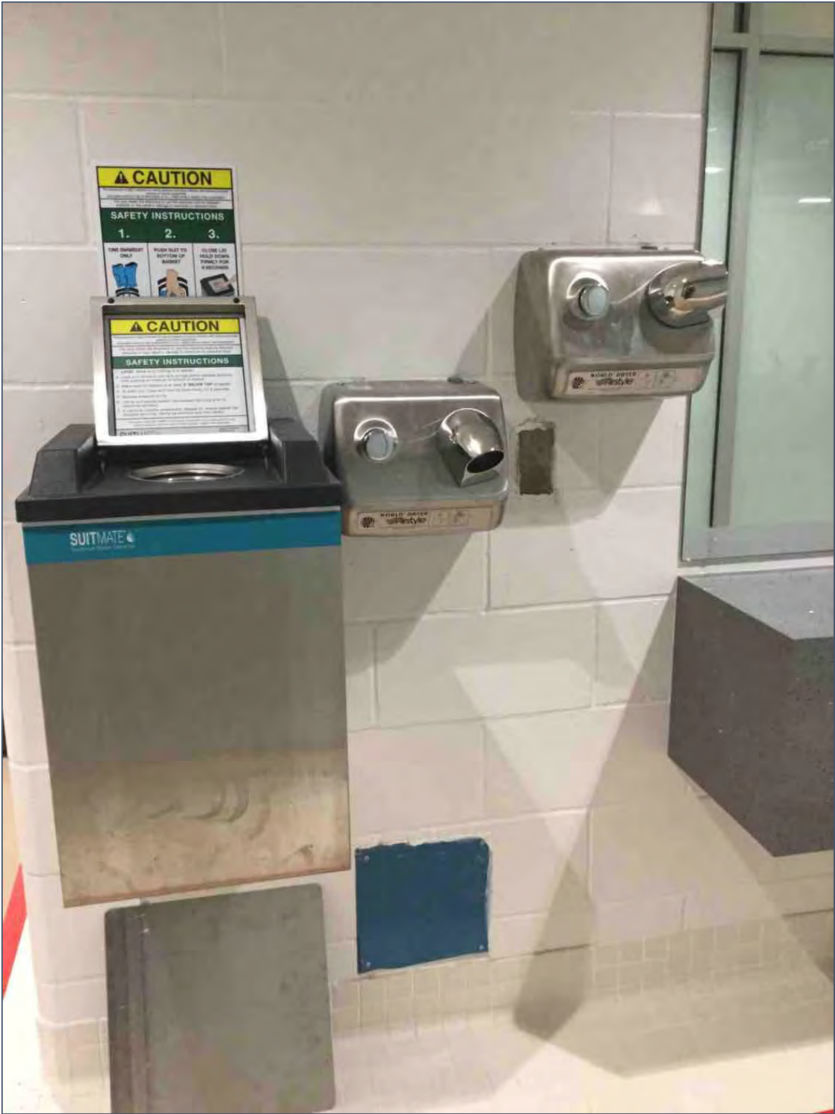
Phase 1C – Dryer install in universal changerroom
