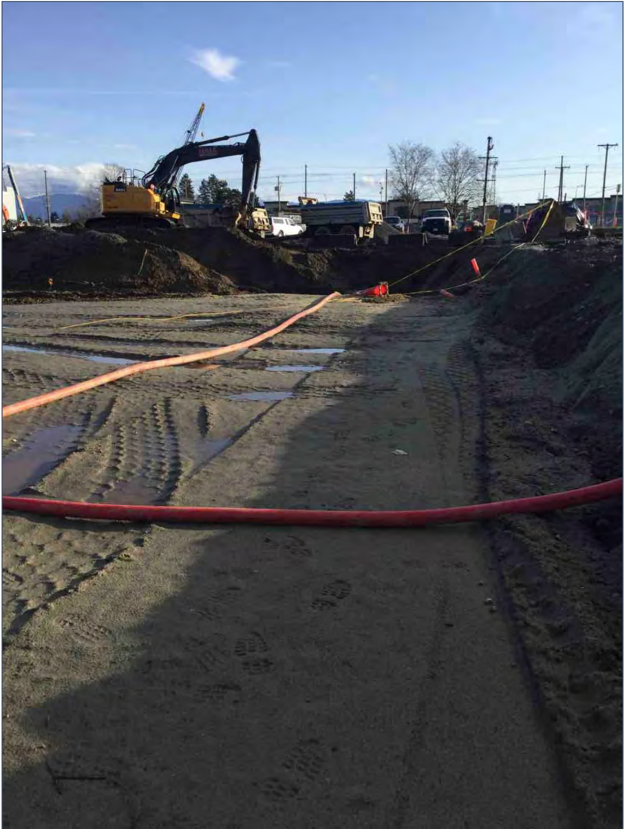
Phase 2 – Bulk excavation
