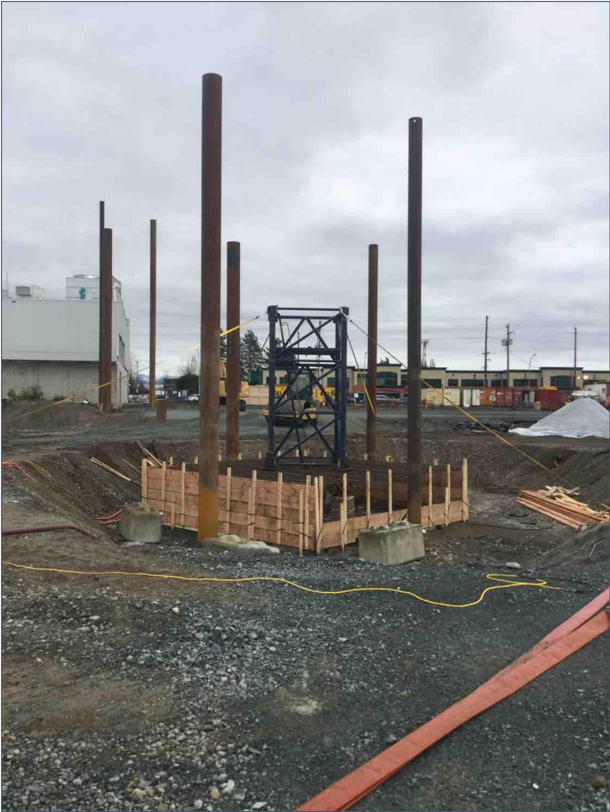
Phase 2 – Crane base
