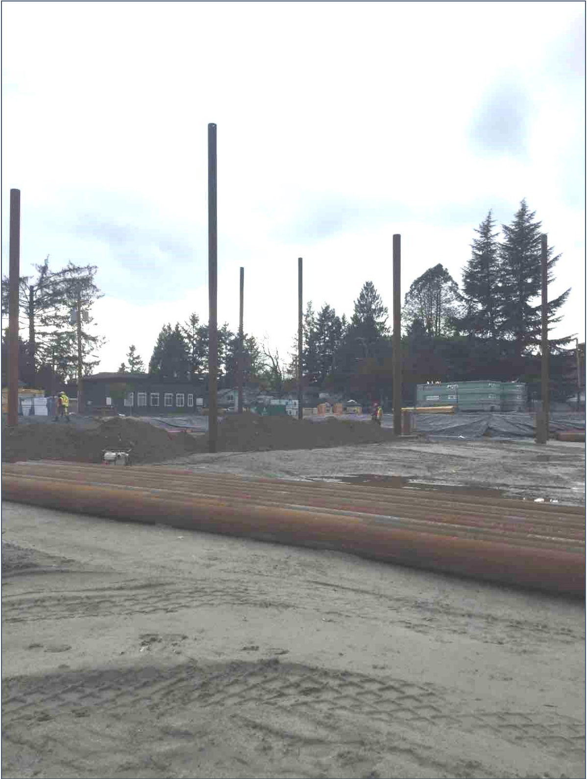
Phase 2 – Piling to SW corner
