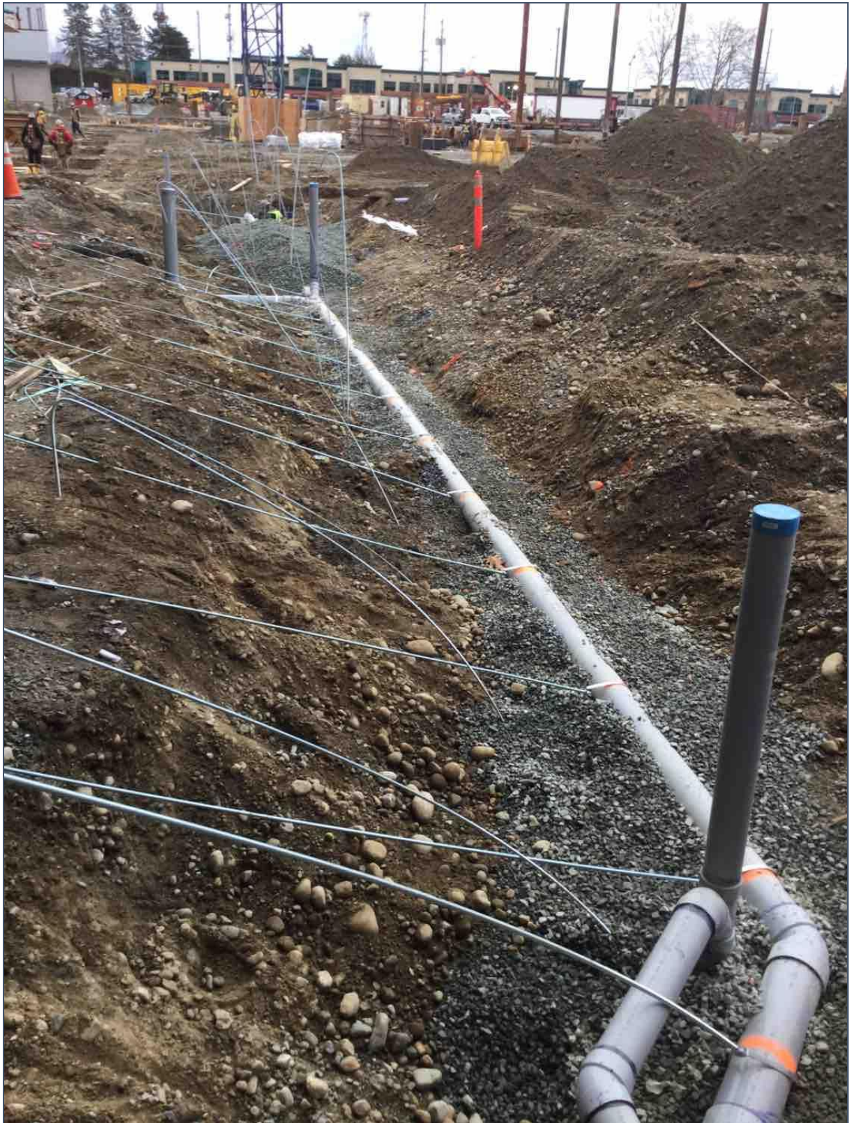
Phase 2 – Under slab drainage
